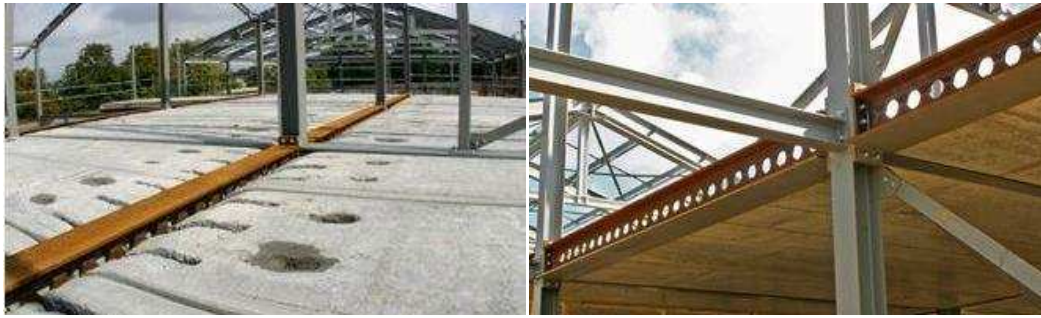
Fig. 1: USFB used with profiled steel decking (top) and with precast concrete unit (bottom) (adopted by [8])
