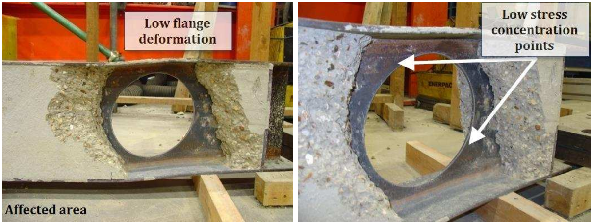
Fig. 14: Failure mode for partially encased USFB No.2 at opening after removal of the damaged concrete
