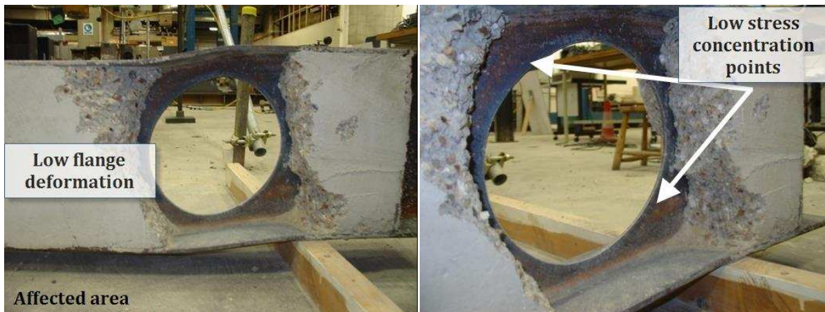
Fig. 13: Failure mode for partially encased USFB No.1 at opening after removal of the damaged concrete
