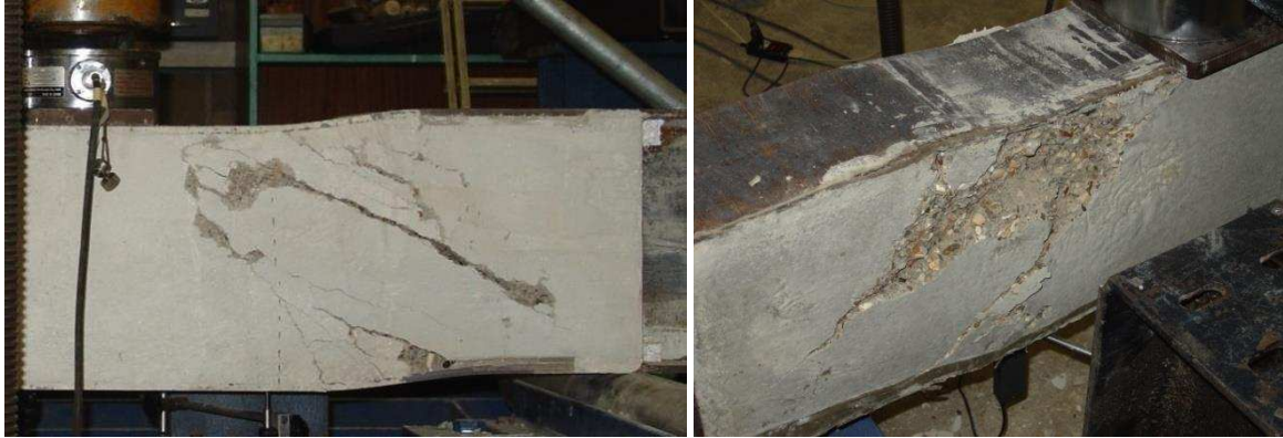
Fig. 11: USFB No.3 with concrete bursting
