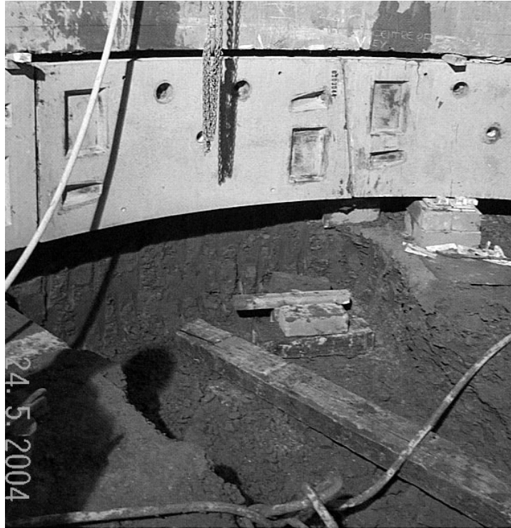
Figure 9 Overdig at position of key segment
