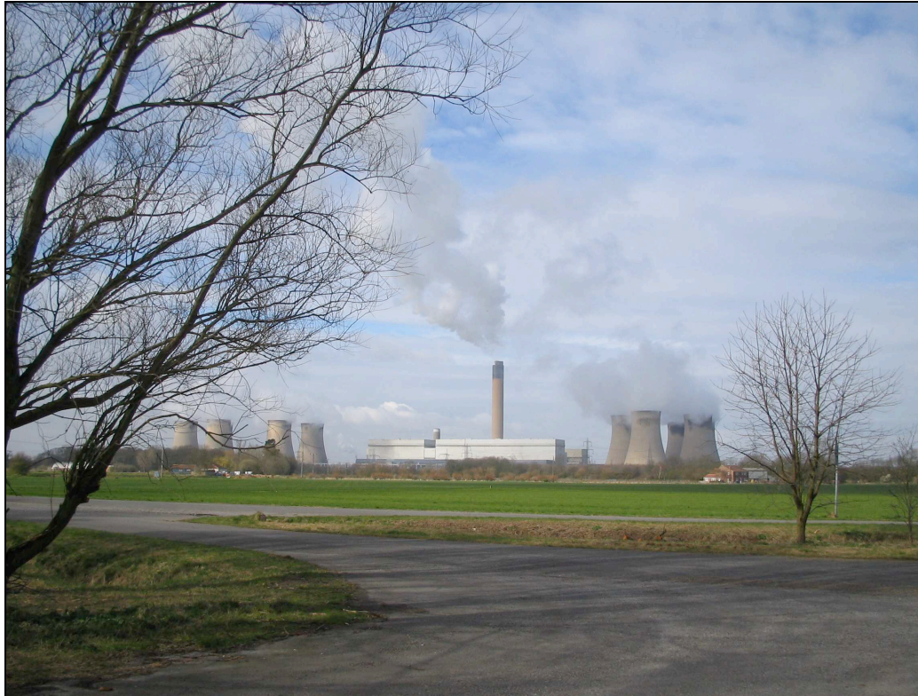
Fig. 2b. Drax coal-fired power station (Photograph taken by first author, April 2008).
