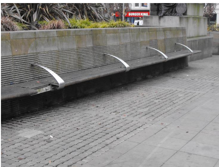
Figure 3: Taller wall, armrest and cobbled paving, Piccadilly Gardens, Manchester
