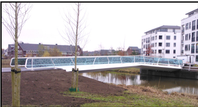
'Bronlibelle' Bridge in Harderwijk, the Netherlands. A 6.3 m wide, 22 m long GFRP bicycle / footbridge connecting two new districts of Harderwijk. At the same time unlocking an efficient route for heavy emergency vehicles (e.g. firetrucks). The bridge deck is made by applying the vacuum infusion technology, thus providing excellent properties with desired freedom for design. The bridge is designed according to CUR96, EN 1990 and EN 1991. Architectural and preliminary design by Royal HaskoningDHV. Engineering, production and installation by Delft Infra Composites B.V.
