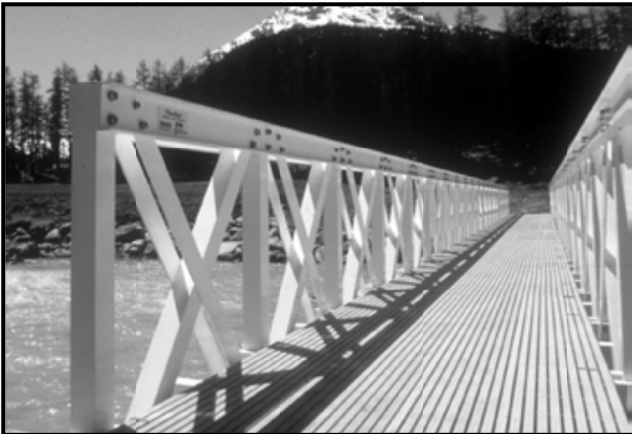
Ponteresina, Switzerland. Footbridge in 2 spans of 12.5 m for temporary use in the winter (designer: prof. T. Keller). GFRP profiles. Contractor: Fiberline Composites A/S, Middelfart, Denmark, 1997.
