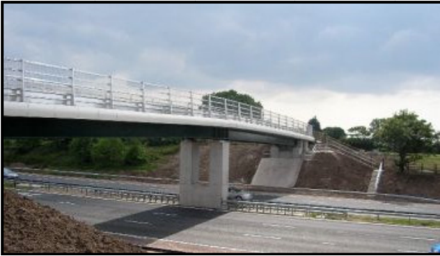
Motorway M6, Lancashire, UK. Road bridge over a motorway. The bridge is 52 m long and has been designed to carry vehicles up to 400 kN weight. GFRP pultruded profiles “FBD 600 ASSET”. Contractor: Fiberline Composites A/S, Middelfart, Danmark, 2006.
