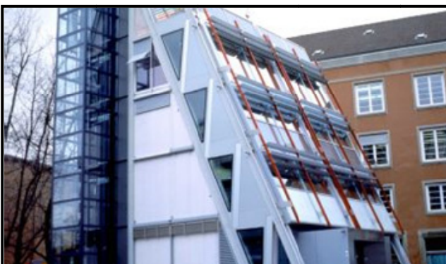
Münchensteinerstrasse, Basilea. Eyecatcher building made of GFRP pultruded beam. The building consists of 5 floors with a total of 15 m of height; the surface amounts to 120 m 2 . Contractor: Fiberline Composites A/S, Middelfart, Denmark, 1999.
