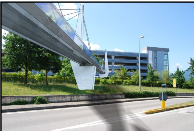
Salerno (Italy). Pedestrian bridge at the University of Salerno. Length: 148 m; main span: 37 m. GFRP pultruded I-beam. The deck is made of GFRP sandwich panels. Designer: prof. Luciano Feo, 2014 (In construction).
