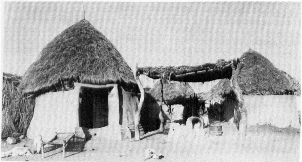
Figure 5-3: Traditional rural mud house in coastal region
