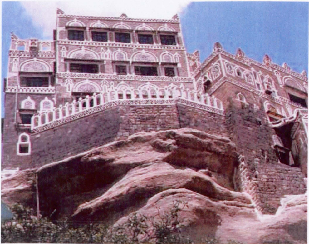
Figure 5-13 Stone used for the ground and first floors while brick for the upper floors.
