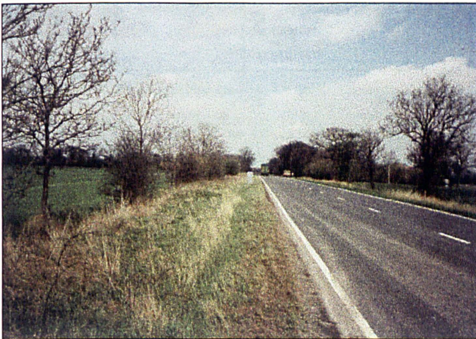
Figure 5-8 View of the straight road section of site 1 (real road)
