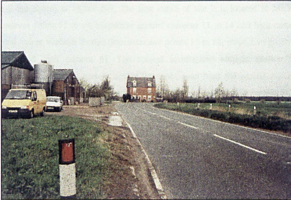
Figure 5-7 View of the curved road section of site 1 – Caville Bends (real road)
