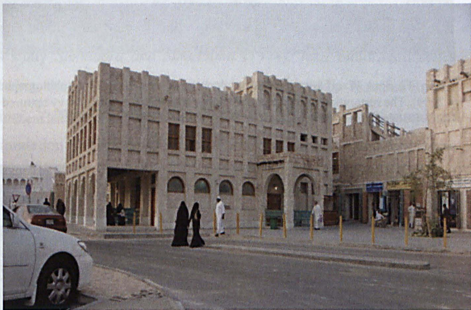
Fig. 11. Souk Waqif after restoration/reconstruction in 2004-2005 using old building materials such as adobe walls and timber doors and window frames, photographed in 2009.
