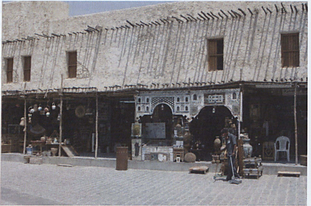
Fig. 12. Souk Waqif after restoration/reconstruction in 2004-2005 (photographed in 2009). The restoration used a primitive adobe material to create a wavy textured wall. Such wooden pillars were used in thatching work. This is how traditional modest Qatari houses would have appeared in the past.
