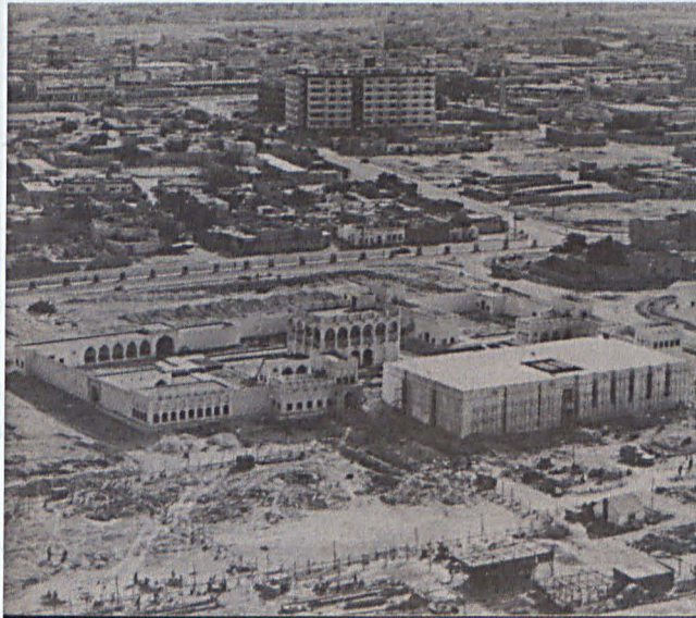
Fig. 28. Restoration work on the Old Emiri Palace and the development of the surrounding area.
