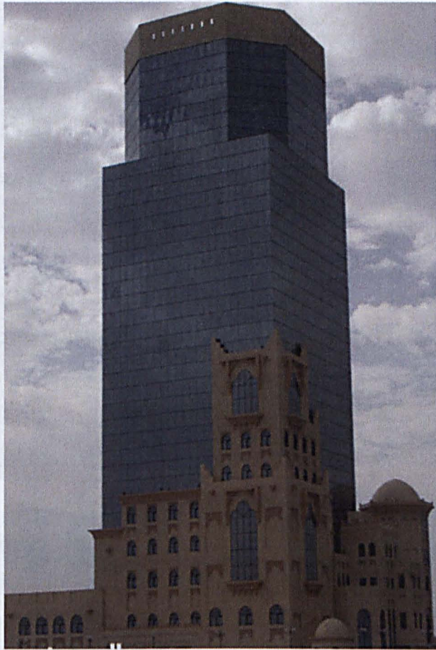
Fig. 16. Barzan Tower, which is located among other skyscrapers on Doha's corniche.
