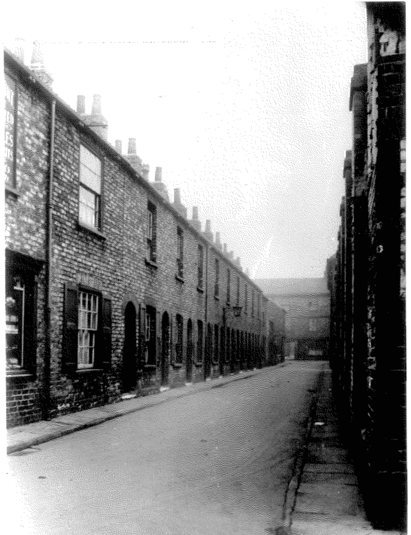
(12) Nos. 6-24 Carmelite Street, off Hungate. Early 1930's. All these were through, two-roomed houses. When inspected in 1935 none contained a sink, and water for each was supplied from an external tap. (See Map 11)
