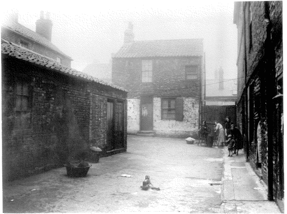
(11) Wide Yard, Hungate, late 1920's. Contained ten houses and tenements, most of which were two-roomed and back-to-back, "dilapidated and unfit." (See Map 11)
