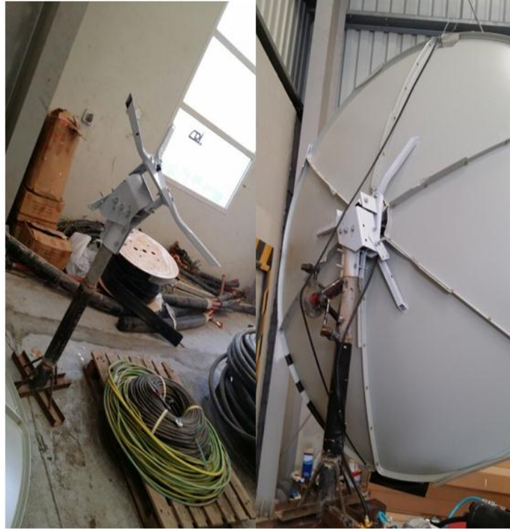
Figure 3.7 4\text{m}^2 parabolic dish with installed long iron base stand
