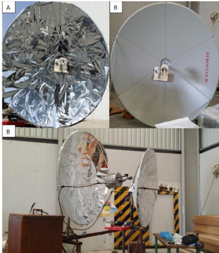
Figure3.8 Both parabolic dishes installed at both ends of long iron base (5 m)
