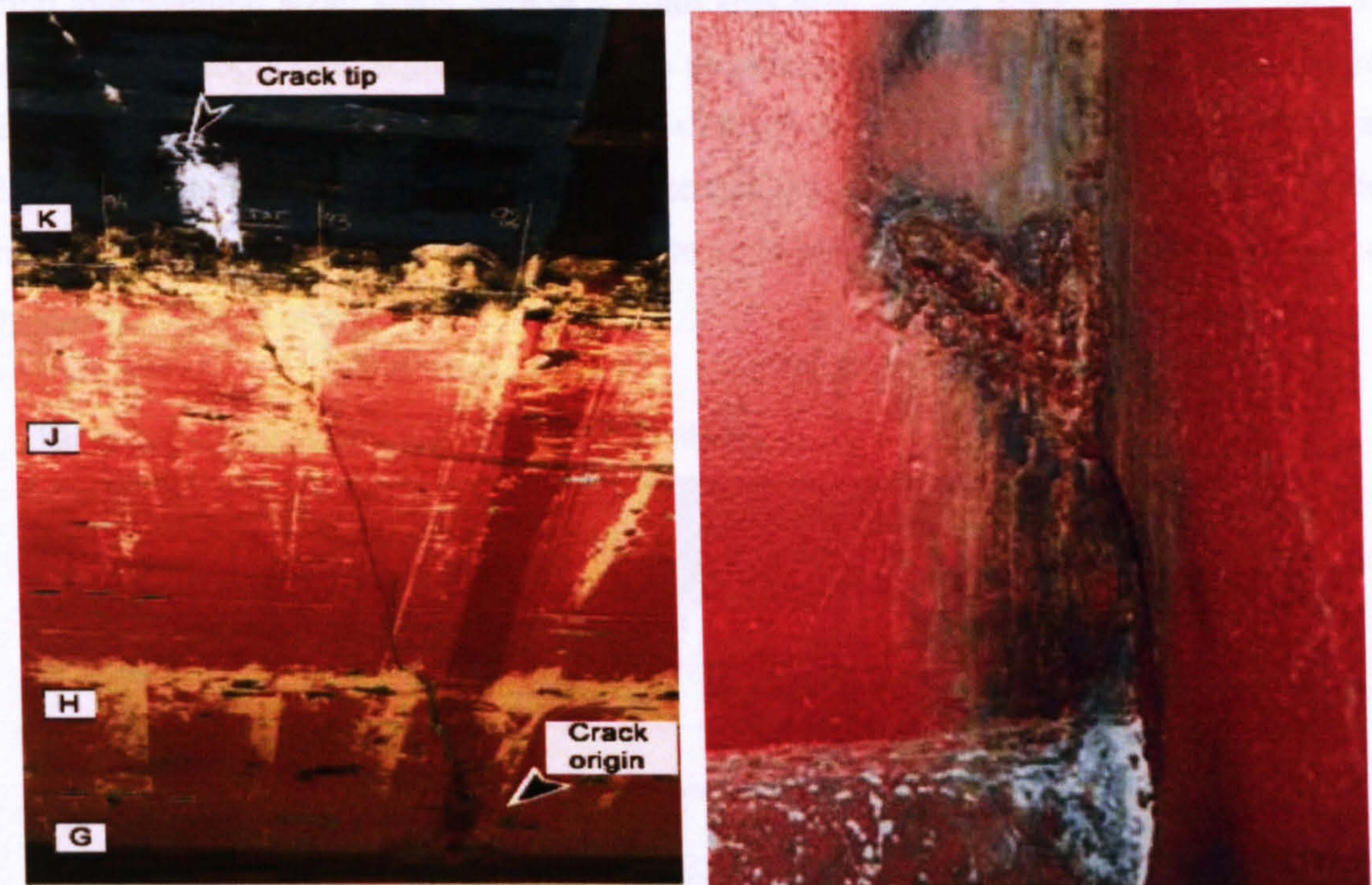
Figure 1.2 – The principal fracture and a fracture from which water ingress was observed.
