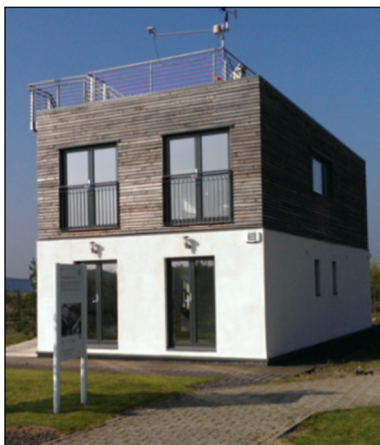
Figure 1: the Applegreen house at the BRE Innovation Park, Motherwell.
