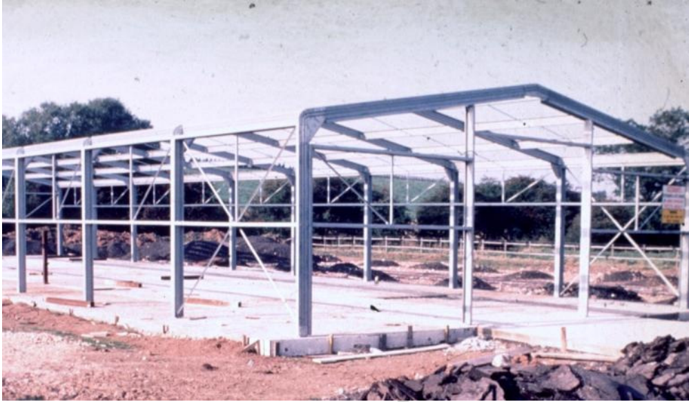
Fig. 1: Cold-formed steel portal framing system
