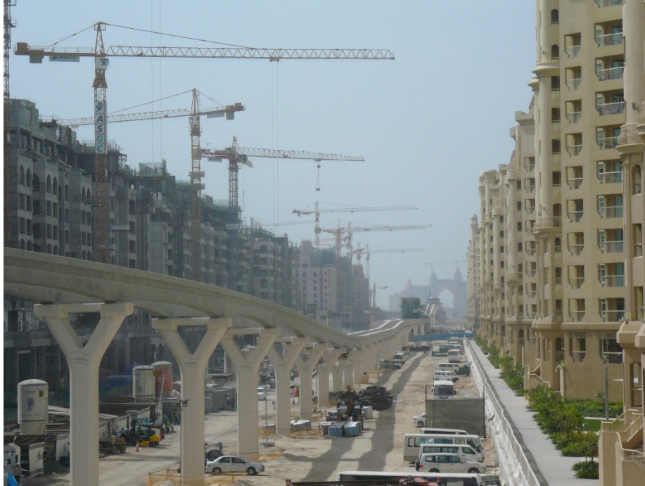
Figure 4: The apartment buildings at the trunk of the Palm Jumeirah under construction in 2008. Source: Authors.
