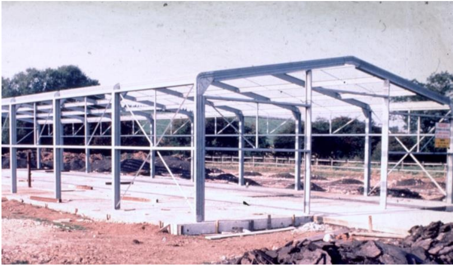
Fig.1 Typical cold-formed steel portal framing system
