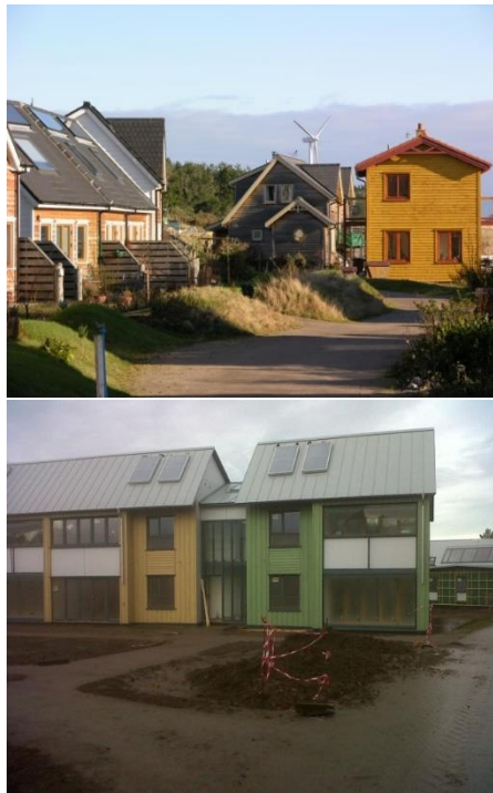
Figure 2 Findhorn village and apartment block (monitoring site)
