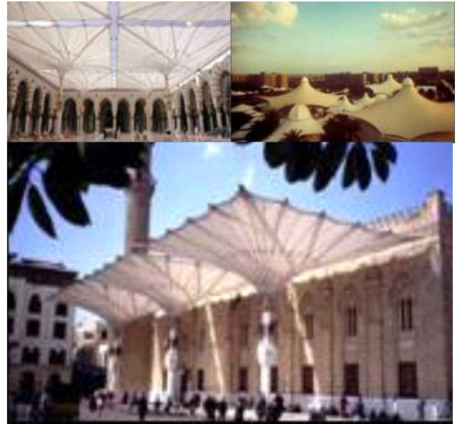
Figure 1. The use of conical membrane structures in different architectural projects (Photo courtesy TENSINET Library [23])
