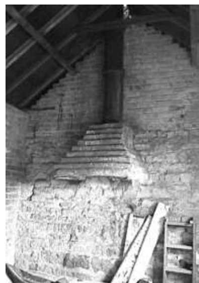
Figure 21: Photograph of the remaining forge chimney
