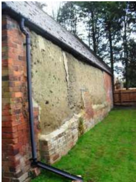
Figure 41: External mud wall of barn
