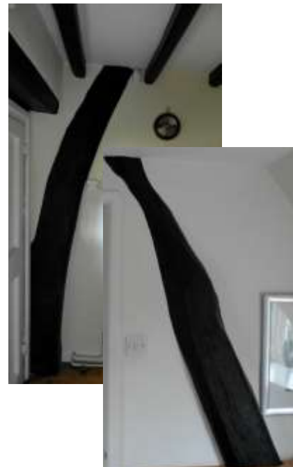
Figure 59: Cruck beams at Tudor House, ground and 1 st floors
