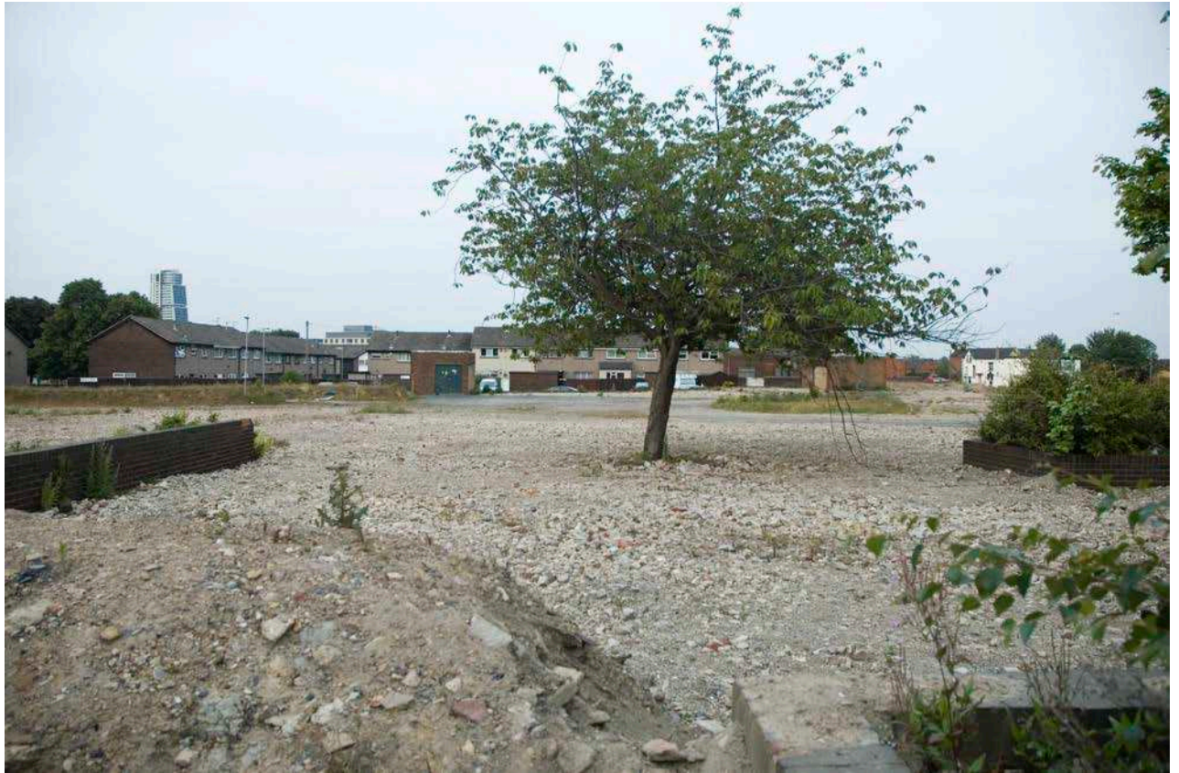
Figure 3.7 Holbeck Towers rubble site
