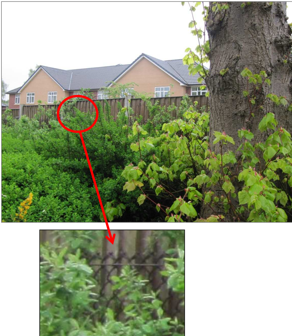
Figure 37 Rear boundary with no trellis added and close up of chain link fencing
