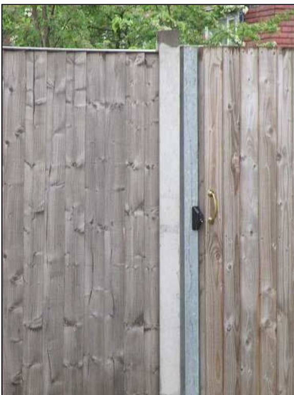
Figure 40 Slam-to-lock on a side gate
