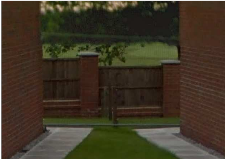
Figure 34 Rear boundary at CIS-2
