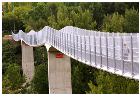
Figure 4. Stress ribbon footbridge in Cuenca, Spain (photo by ACCIONA [19]).
