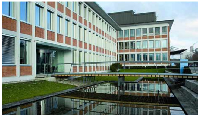
Figure 1. Empa bowstring arch footbridge [14]. Reprinted with permission from ref. [14]. Copyright 2009 Empa.
