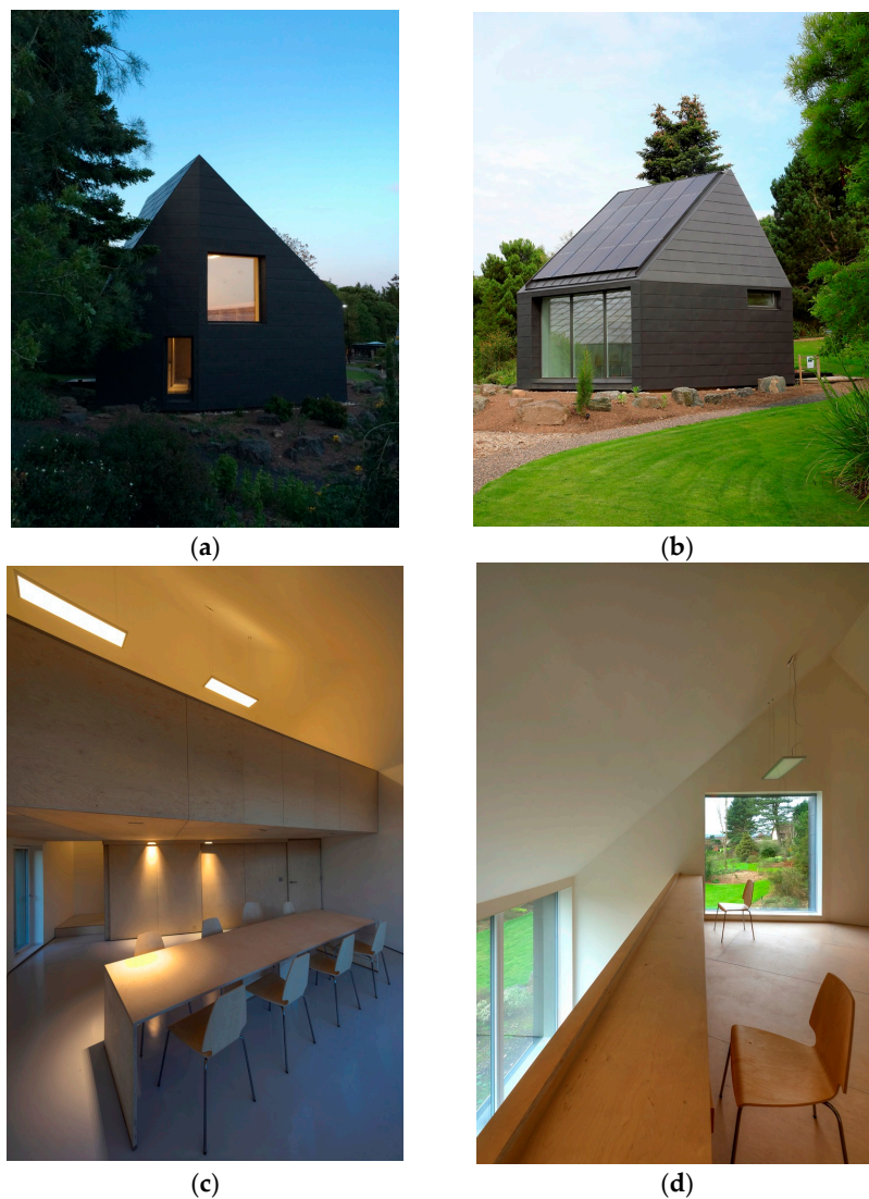
Figure 2. (a) West elevation; (b) South east elevation; (c) Ground floor space; (d) First floor space.
