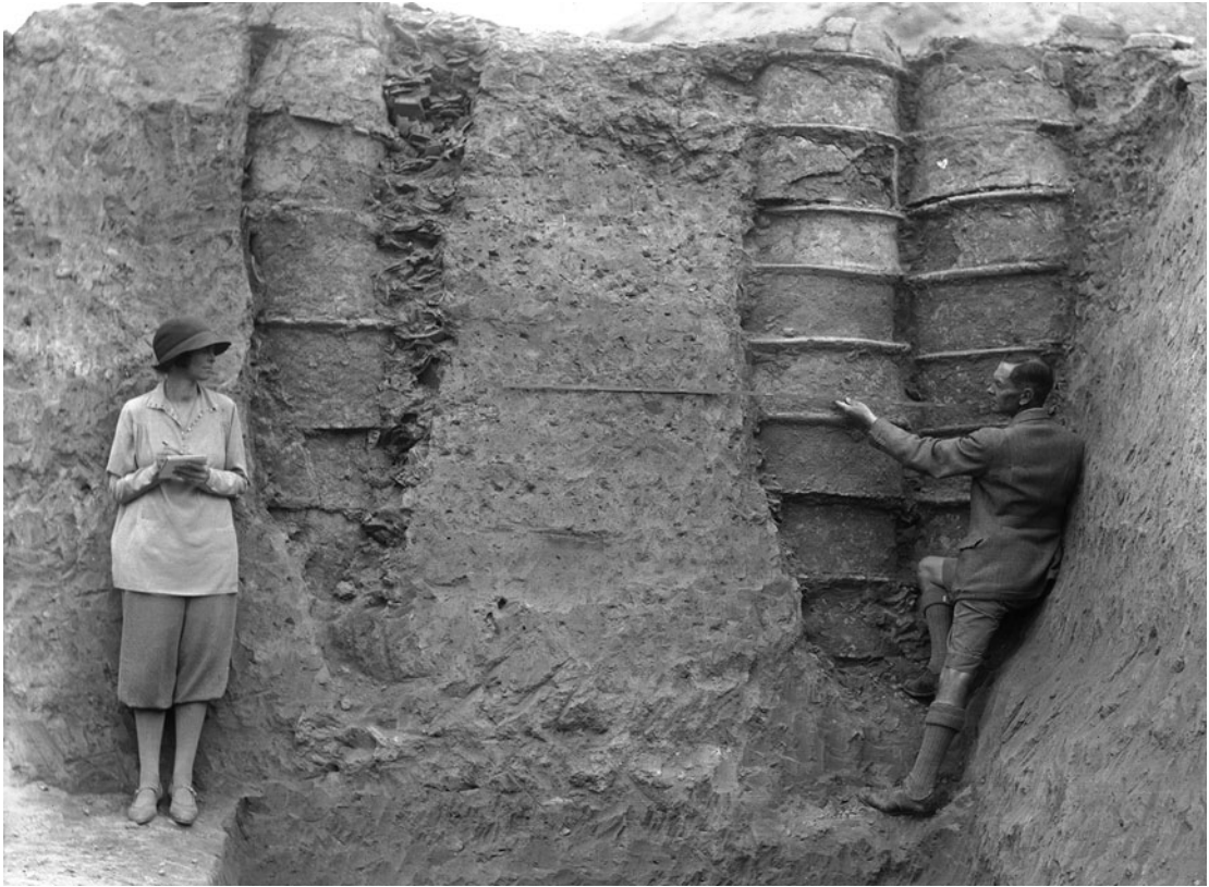
Fig. 6 Leonard and Katharine Woolley at Ur, with ring-drains in situ (photograph BM-Ur-GN-1592 reproduced by permission of the Trustees of the British Museum). Clearly visible, between the wall of the left-most drain shaft and the ring-drain itself, is the usual packing with potsherds to improve drainage
