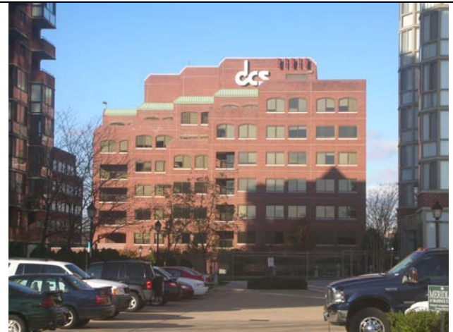
West – Braddock Place Office Building
