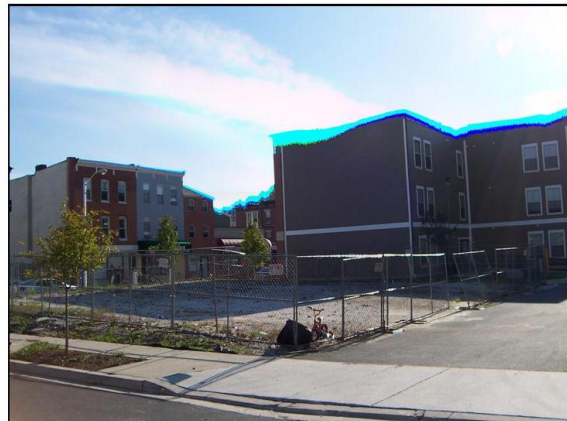
Rear view of subject with ingress / egress
