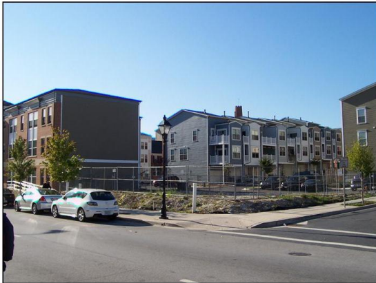
Hard Corner of Subject Property
