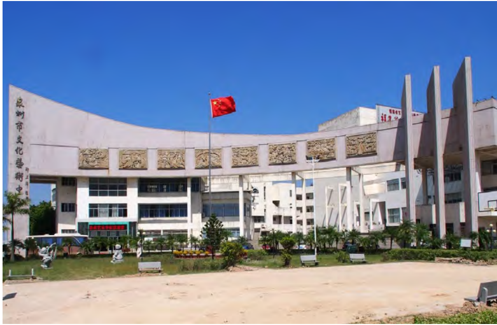
Fig. 6.1 Fujiansheng Quanzhou Yishu Xuexiao [Fujian Province Quanzhou Arts School] (field photo 2013)
