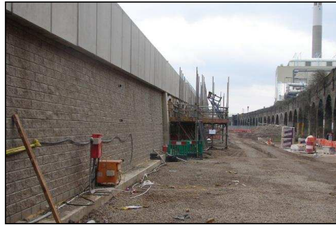
Figure 10: SS408 (Reinforced earth structure)
