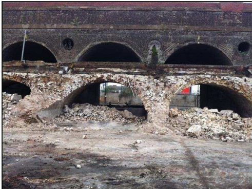
Figure 3: Bay Viaduct (part demolished) (Skanska)
