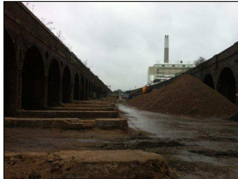
Figure 4: Demolished Bay Viaduct and crushed brick stockpile (Skanska)
