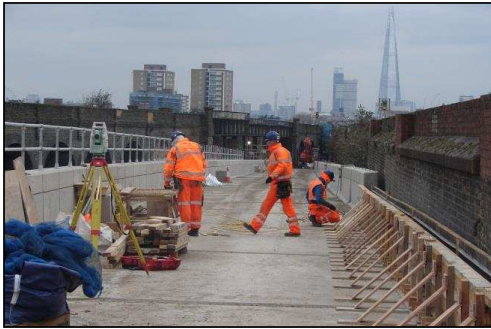
Figure 9: SS408 (Reinforced earth structure)
