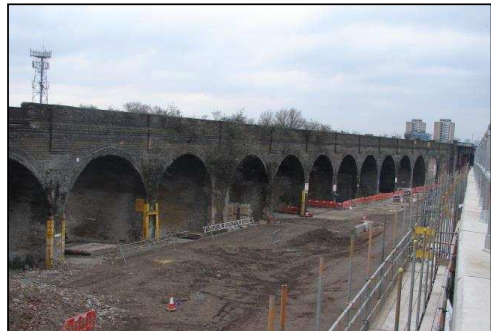
Figure 8: New Cross Loop Viaduct (to be demolished)
