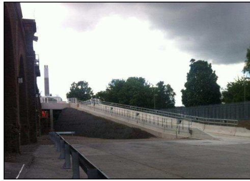
Figure 6: Completed RRV2 (Skanska)
