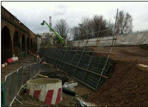
Figure 5: RRV2 under construction (with crushed brick fill) (Skanska)
