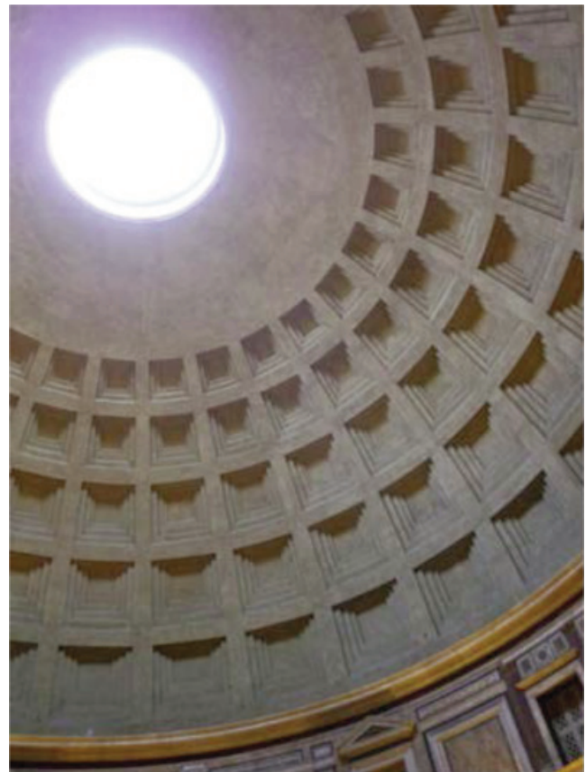
Figure 1. The concrete roof the Pantheon, Rome.
