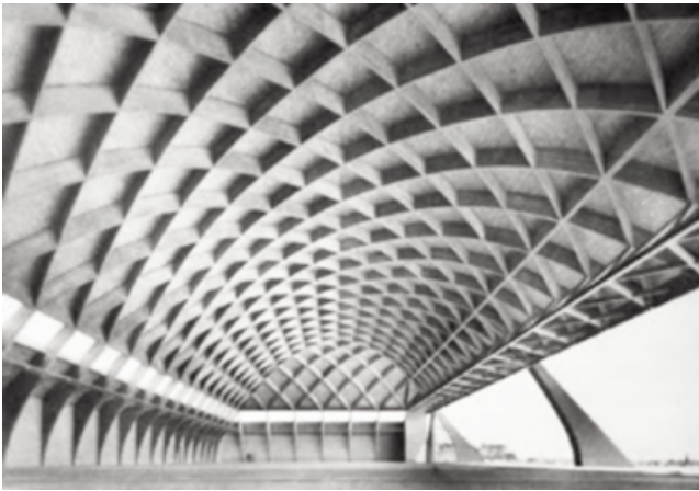
Figure 2. Aircraft Hangars at Orvieto Airport by Pier Luigi Nervi (1935–1938, 1939–1942).
