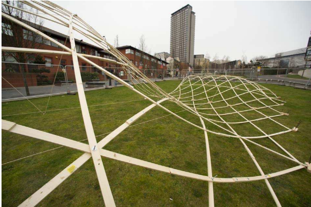
Figure 1. The swells of the timber gridshell structure against the backdrop of Sheffield
