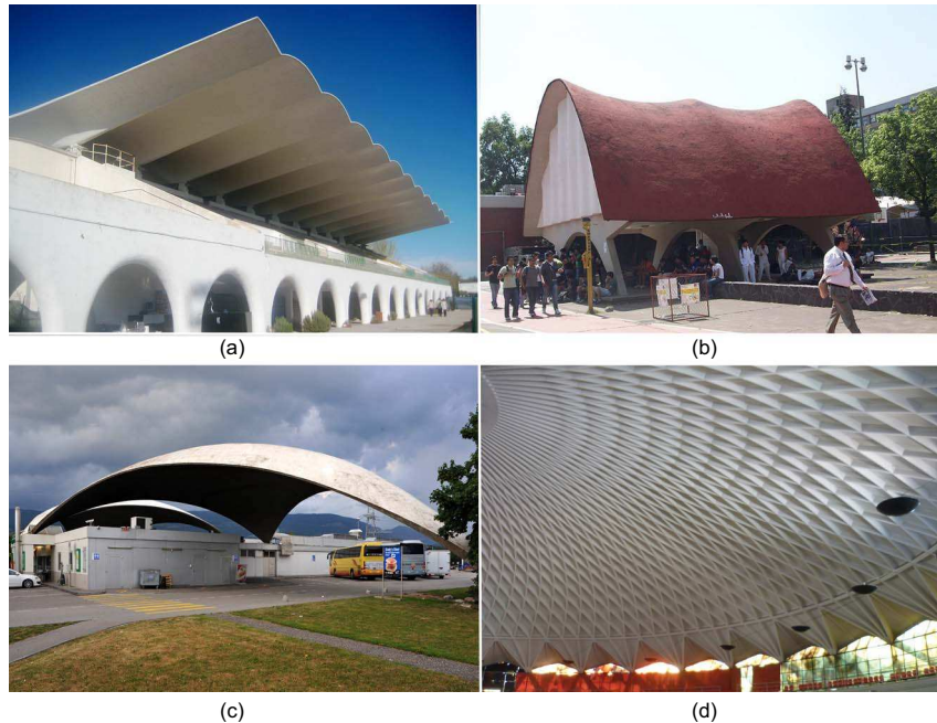
Figure 4. (a) Thin repeated concrete shells form the canopy of La Zarzuela Hippodromo roof by Torroja [By Outisnn (Own work) (GFDL ( http://www.gnu.org/copyleft/fdl.html ))), via Wikimedia Commons]. (b) Cosmic Ray Pavilion, Mexico City by Felix Candela (1951) [By GAED (Own work) [Public domain], via Wikimedia
