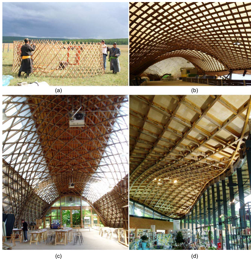
Figure 2. (a) Deployable timber lattice mats are used in the construction of yurts by nomadic tribes in Mongolia. [By Aloxe (Own work) (GFDL ( http://www.gnu.org/copyleft/fdl.html )), via Wikimedia Commons]. (b) The Multihalle at Mannheim, Germany
