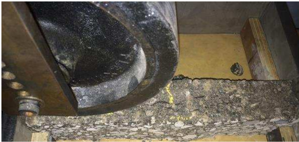
Figure 6-7: Onset of Longitudinal Cracks on 80mm CAEM Base Layer
