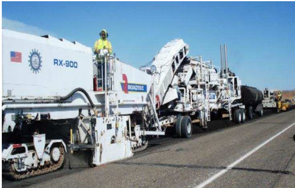
Figure 2-5: Cold in-place recycling train (Roadtec, 2015)
