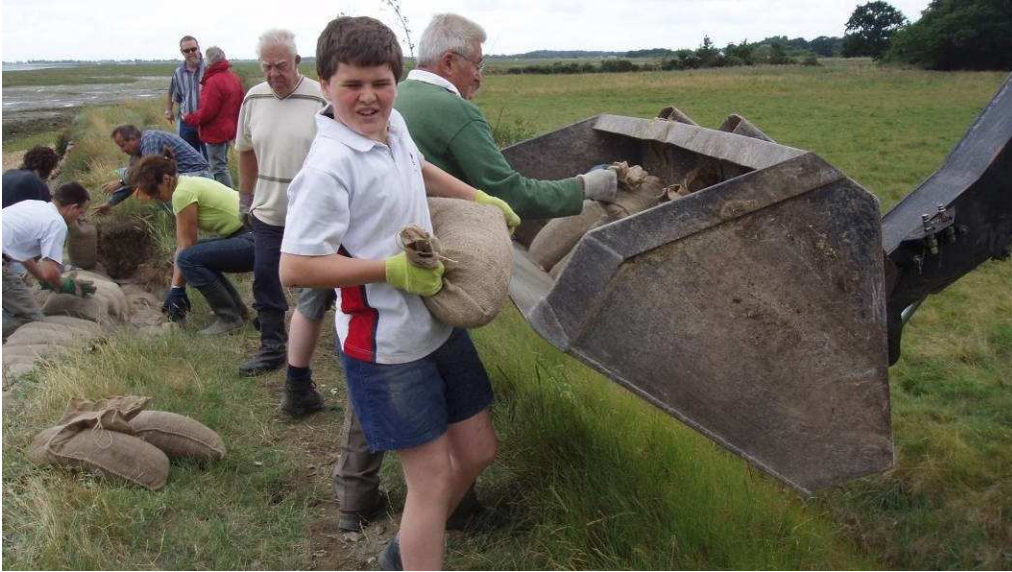
Figure 4-20 Volunteers on crest of sea wall unloading bags from mechanical handler bucket and placing bags (background) 18 July 2009
