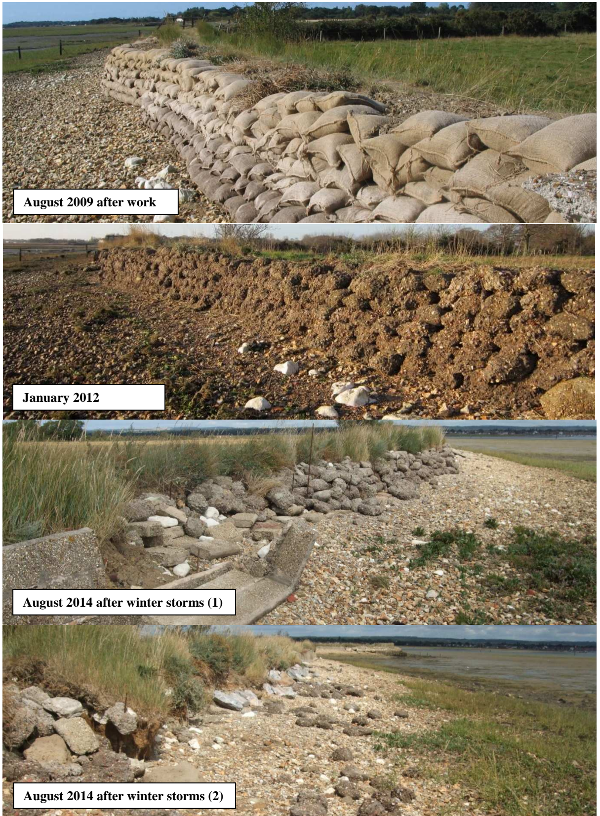
Figure 5-5 Section (B) of Northney Farm sea wall: 2009 to 2014
