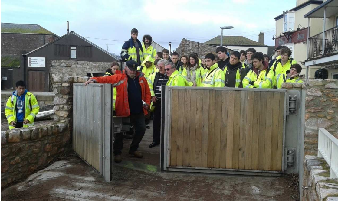
Figure 4-1 Flood gates installed in Teignmouth in 2013
