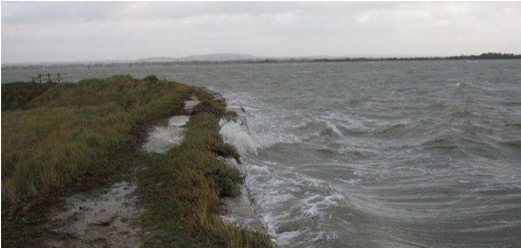
Figure 4-29 Sea conditions at Northney seawall 14 th November 2009 (Courtesy Judy Clark) Notes on conditions: Pressure 998mb; high tide nominal height +4.7m CD/ +2.0m OD, actual maximum water level about + 2.5 to 2.6m OD. i.e. at least 0.5m storm surge.
