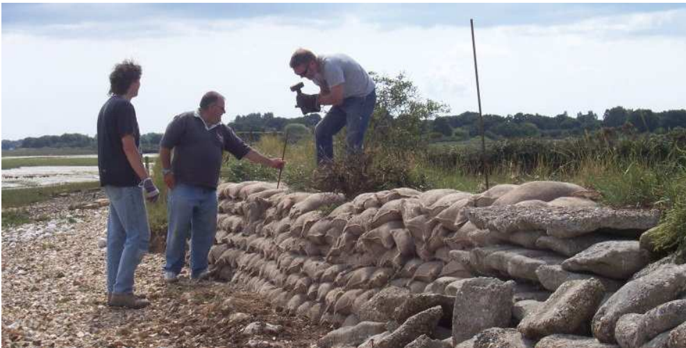
Figure 4-21 Driving steel connector rods through placed sand bags 31 July 2009
