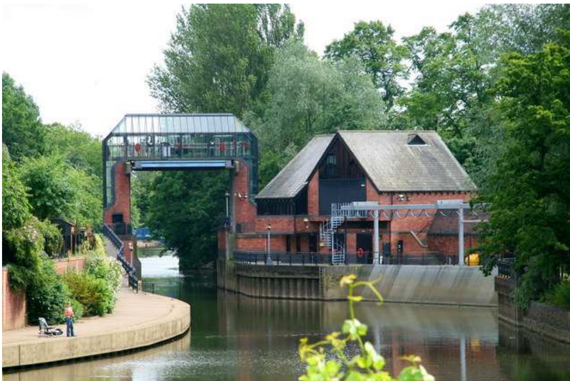
Figure 7-3 The River Foss Barrier as viewed from Castle Mills Bridge, York. (© Copyright David Rogers and licensed for reuse under a Creative Commons Licence. Downloaded 15 th July 2011 from www.geograph.org.uk/photo/866662 )
