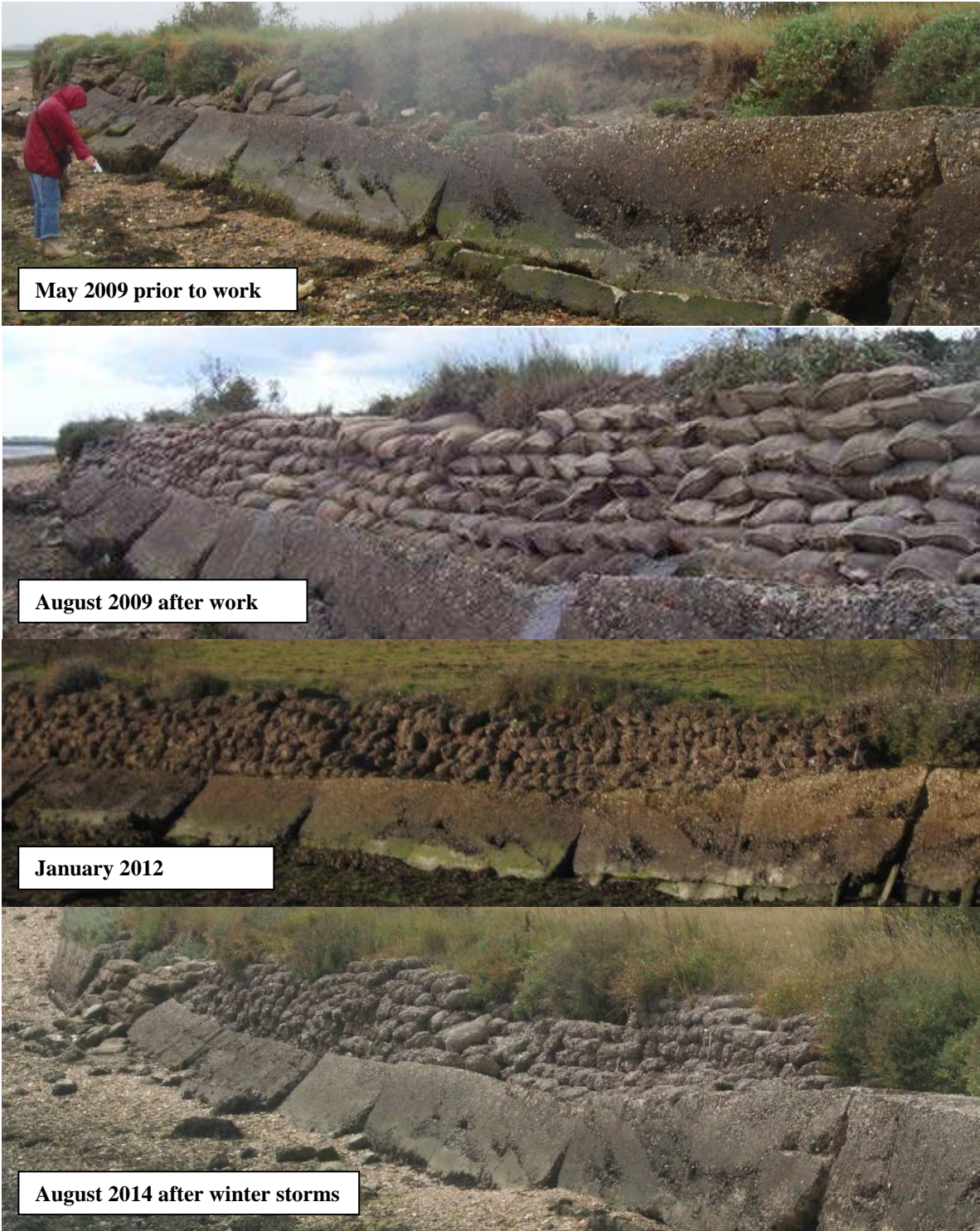
Figure 5-4 Section (A) of Northney Farm sea wall: 2009 to 2014
