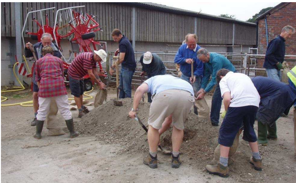
Figure 4-19 NEHRA volunteers filling hessian bags with dry concrete mix 18 July 2009
