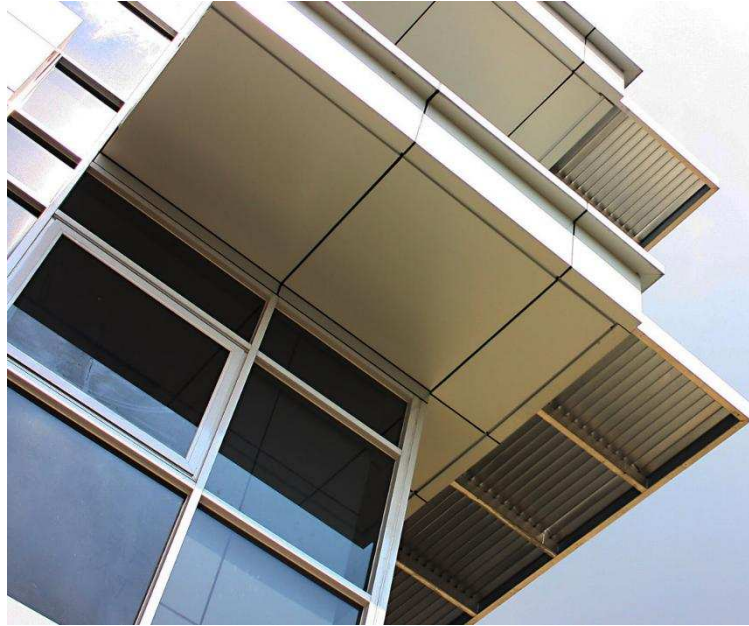
Figure 2.3.15 An application of the solar louvre system on a building (Citytrade, 2015)
