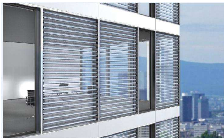
Figure 2.3.6 Building integration of array of solar thermal collector on a green office building (Bine, 2015)
