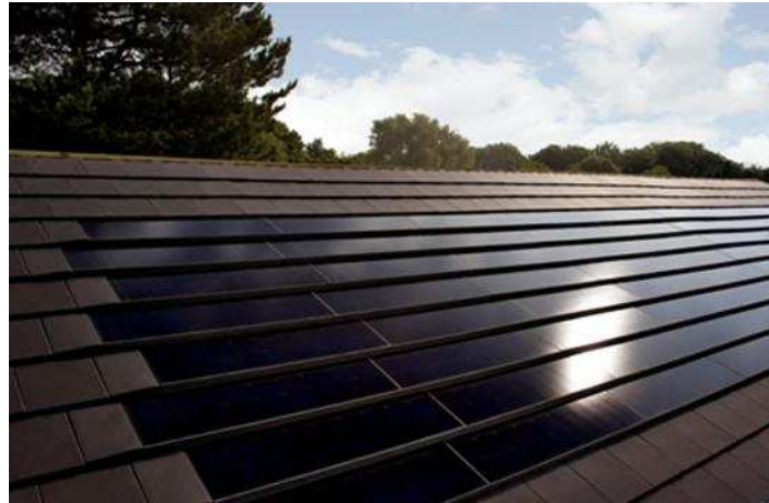
Figure 2.2.17 Photographic view of a PV/T clay roof tile (Building services, 2015)
