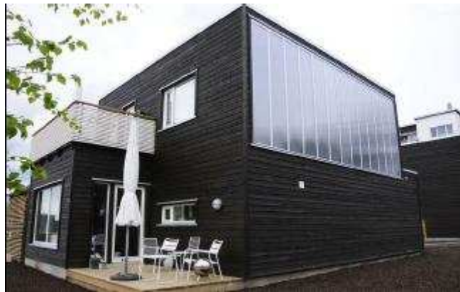
Figure 2.3.13 Building integrated polymeric solar thermal collectors, passive house in Rudshagen, Oslo (IEA-SHC, 2015)
