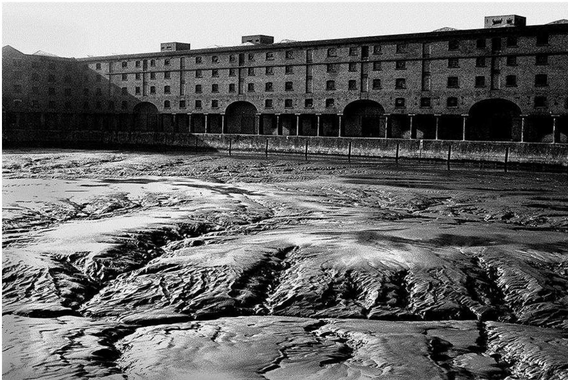
Figure 5. 11 \ The Albert Dock 1981, this picture shows the state of dereliction of the Albert Dock before the regeneration Source \ picture was taken by Photographer Matt Reardon (1981), Liverpool Forum Archive, http://www.yoliverpool.com/forum/showthread.php?108121-Liverpool-s-Albert-Dock-Unseen-1981-Black-and-White-Images-Taken-by-18-Year-Old-Photographer-Matt-Reardon&highlight=albert+dock [Accessed 5 th February 2014]
