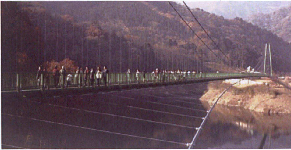
Figure 2.6: The Maple Valley Great Suspension Bridge (MVB), Japan, after [4].
