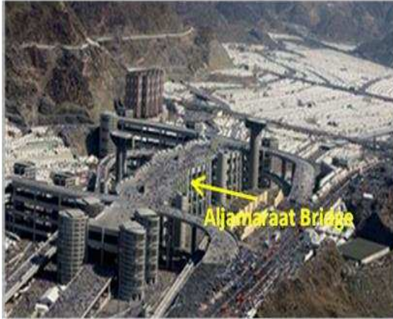
Figure 8.6 (a) Aljamarrat Bridge
