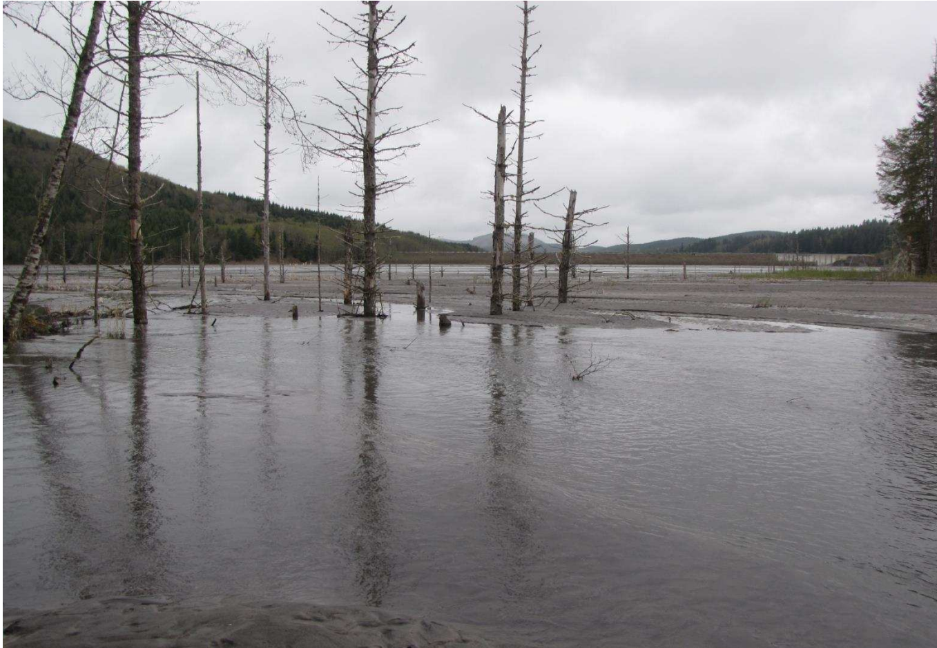
Figure 7.6 Sediment accumulation at the mouth of East Pullen Creek caused by construction of the SRS. The SRS is visible in the middle distance. Photograph by Colin Thorne (2013).
