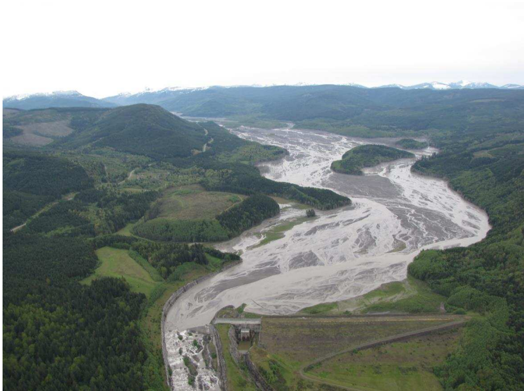
Figure 2.14 North Fork Toutle River Sediment Retention Structure in its Phase 2 operating condition, May 2009. Note the lack of settling pool and the flow passing over the spillway to the left of the structure. Photograph by Colin Thorne (2009).
