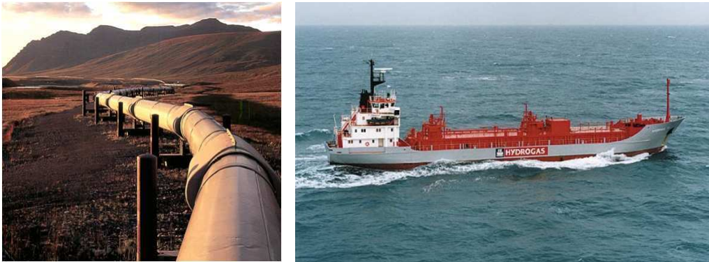
Figure 1.4: The two methods of transport in the CCS process: pipelines (left, [39]), and shipping (right, [26]). Note that most CCS pipelines will be buried below ground. Given the relative lack of CCS pipelines currently, the picture on the left is actually an illustration of an oil pipeline.
