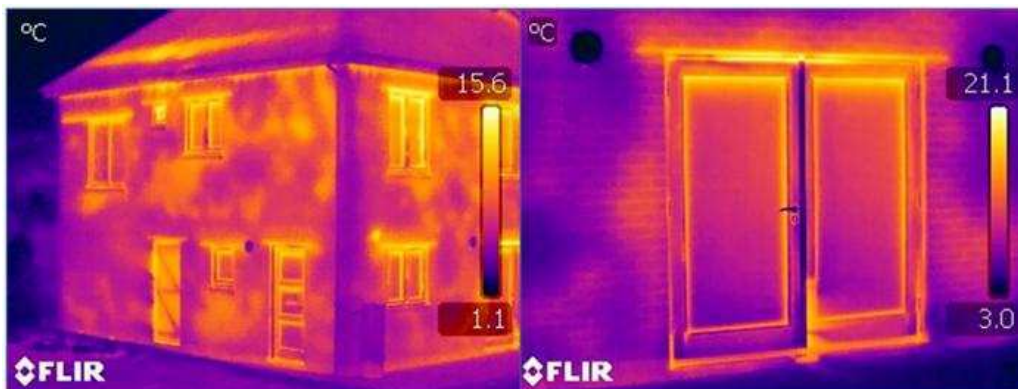
Figure 5-3 - E.On House - Air Leakage Thermal Imaging
