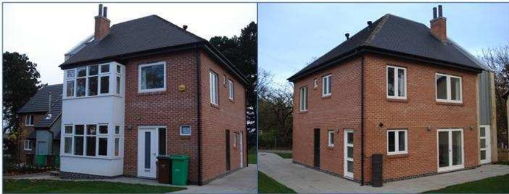
Figure 5-2 - The E.On 2016 Research House
