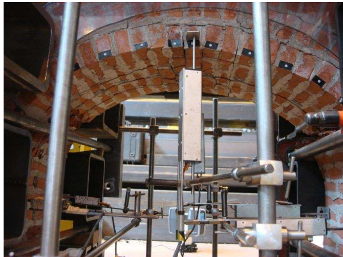
Figure 3.21 Crack failure under uniform load
