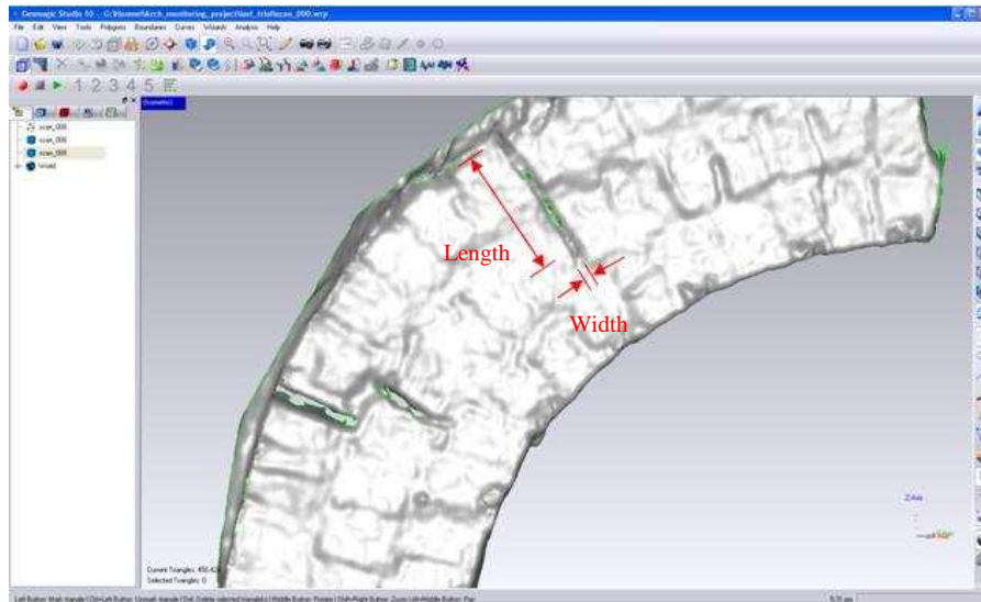
Figure 3.35 Crack width and length measurement
