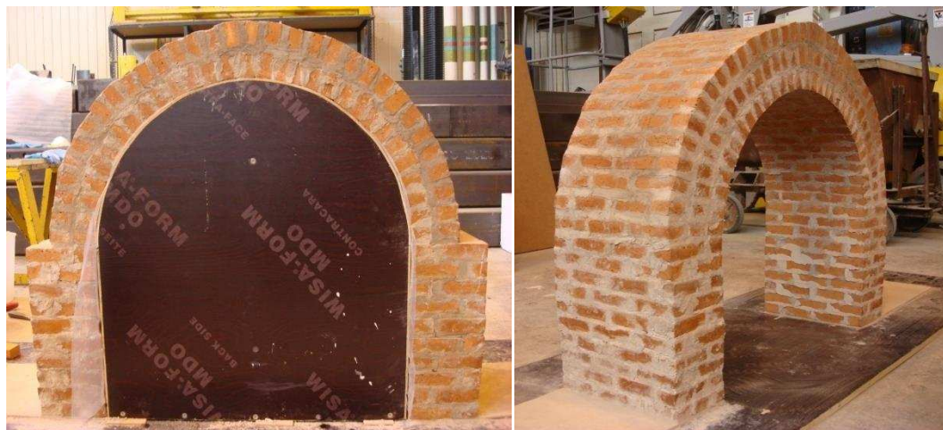
Figure 3.6 (a) Building process with wood arch support; (b) The small-scale brickwork liner of the tunnel
