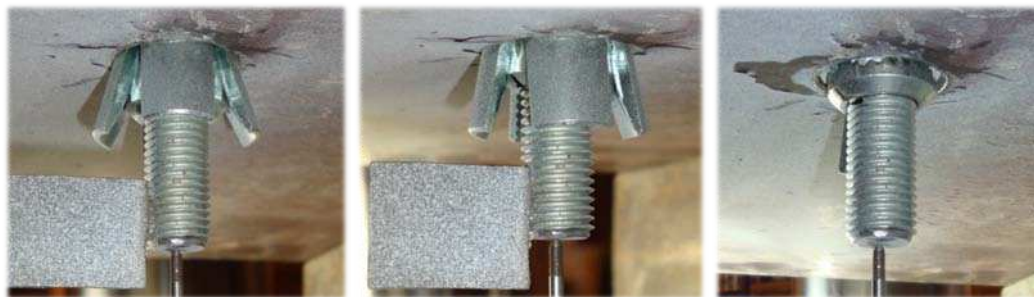
(a) at tightening stage
