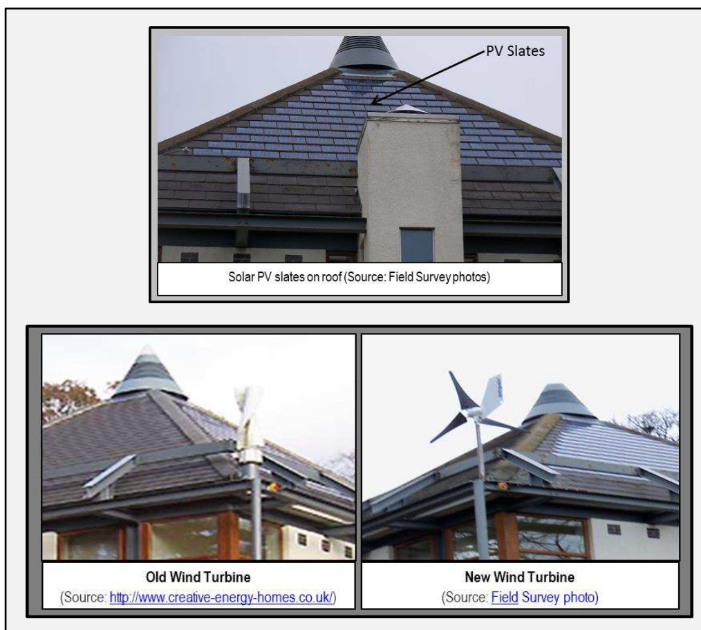
Figure 6.10: David Wilson Millennium Eco-House showing PV slates, the Old and New Wind Turbine
