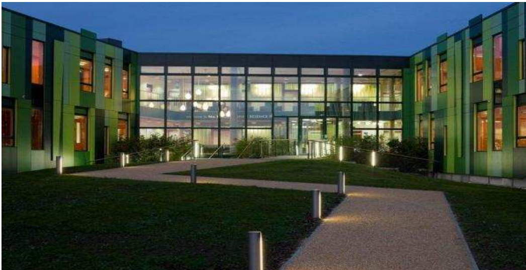
Figure 7.1: The Main Entrance View of the No.1 Nottingham Science Park
