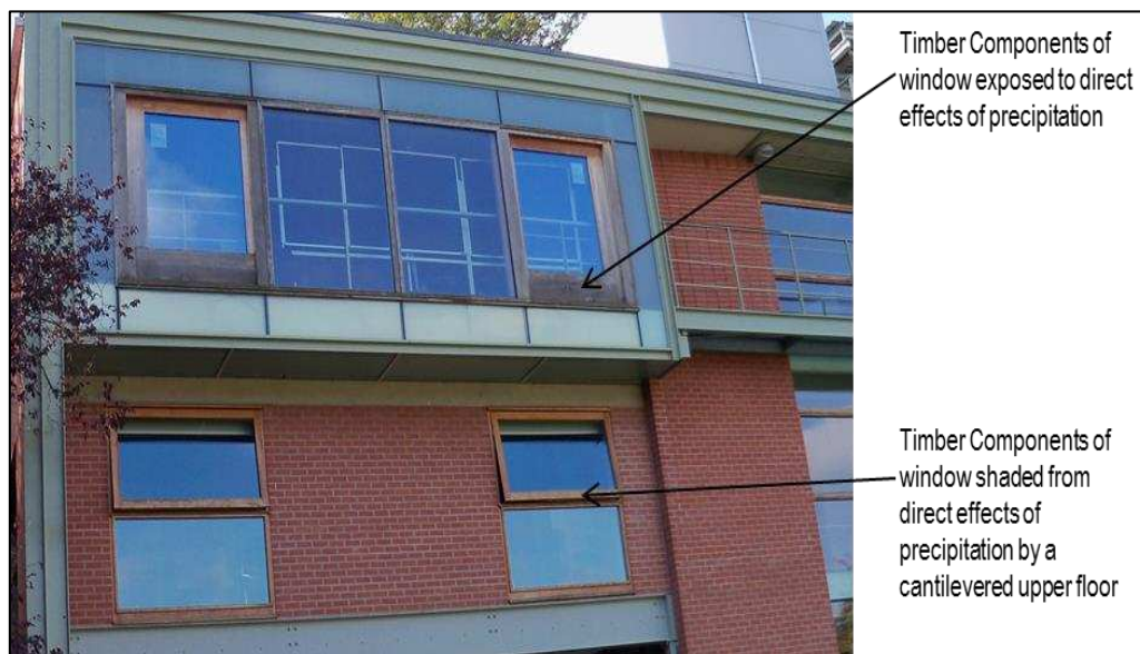
Figure 6.13: Sustainable Research Building (SRB) Showing two different ways timber was used and the resultant effects
