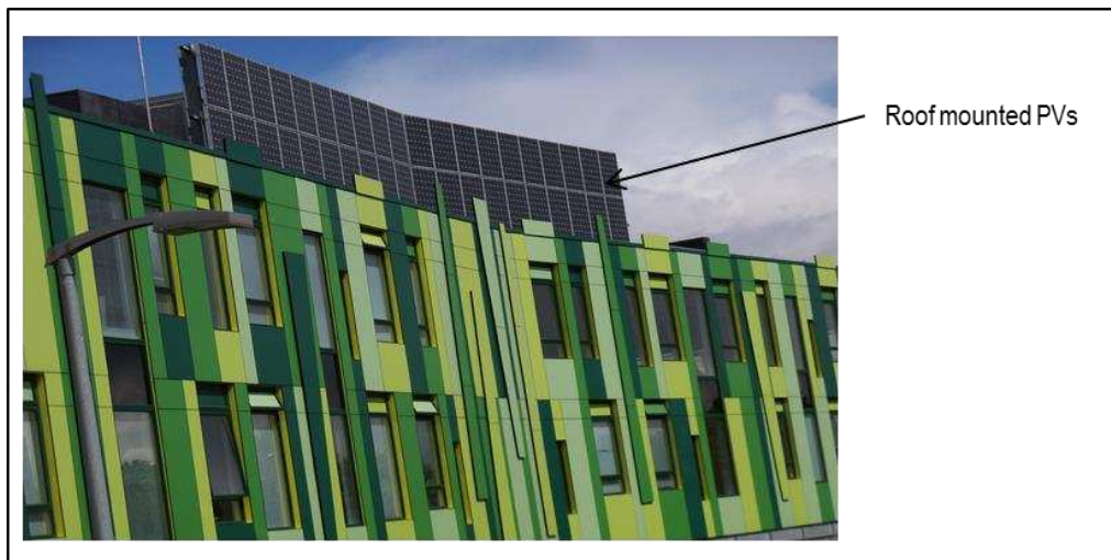
Figure 7.4: Showing the inclination of the Roof Mounted PV Panels
