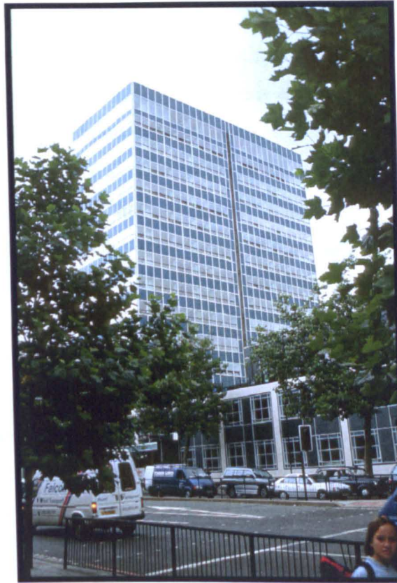
Figure 5.9: Retaining the look. The conversion of the former headquarters of Marathon Oil, Marylebone Road, London into 106 residential units for Berkeley Homes.
