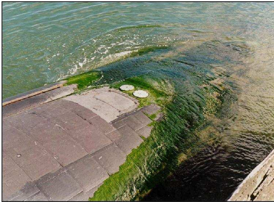
Figure 1.10. An example of Ulva spp. biofouling. Ulva spp. colonisation causing a blockage of an effluent pipe ( figure sourced from Callow and Callow, 2002).
