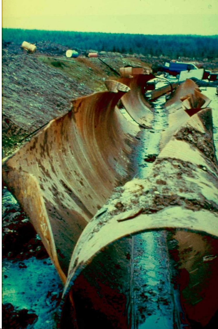
Figure 1.2 Photograph showing a weld failure in a high pressure gas pipe (Photograph courtesy of Advantica PLC.)
