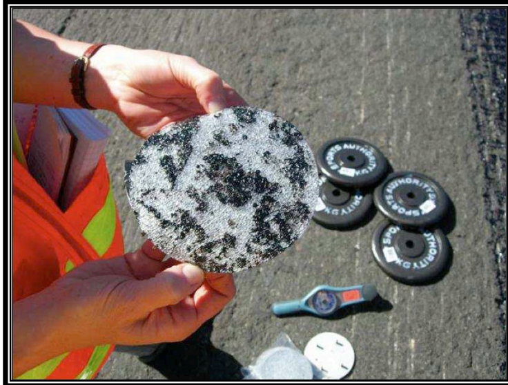
Figure 2.32 Area of coverage of tack coated surface at low temperature (Source: Tandon & Puentes 2006)
