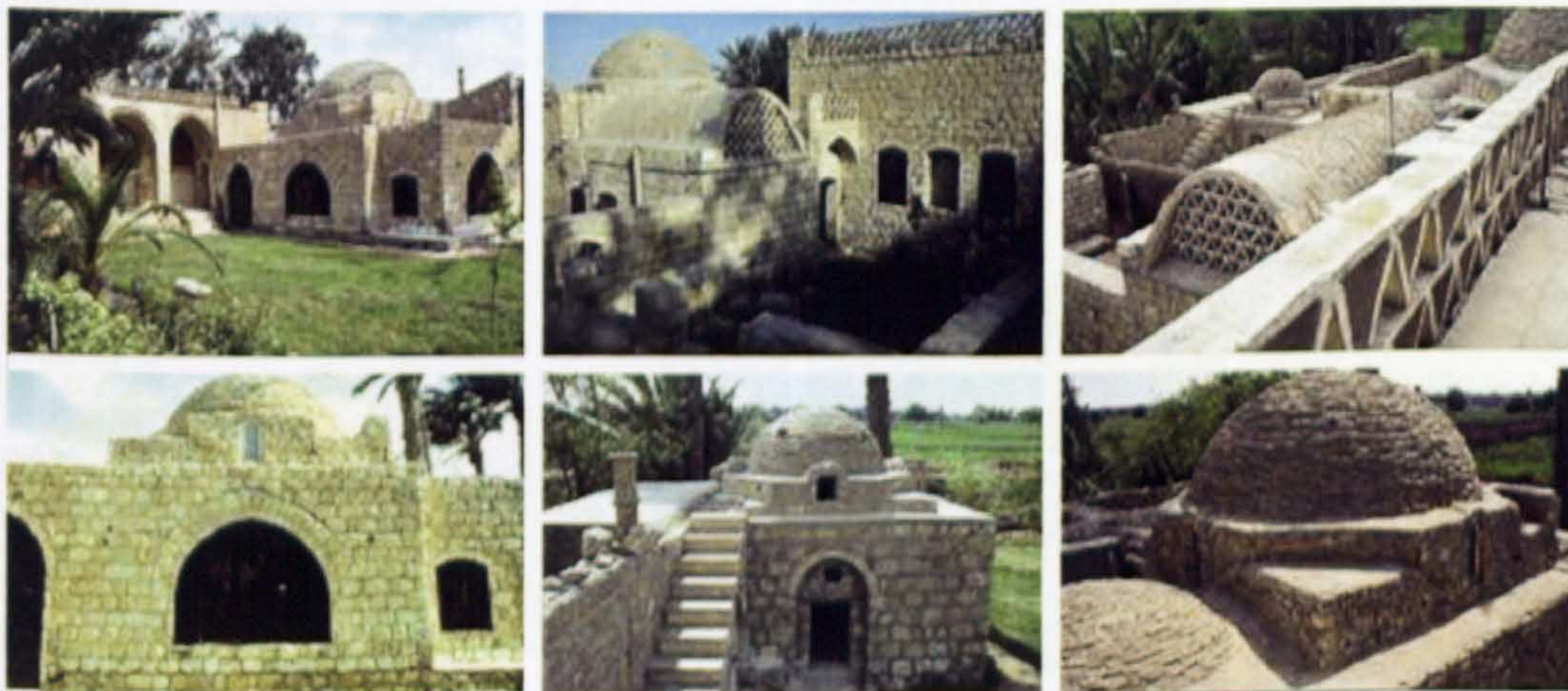
Figure 4-18 Fouad Riad House Roofing Systems, Source: ArchNet Digital Library [13]
