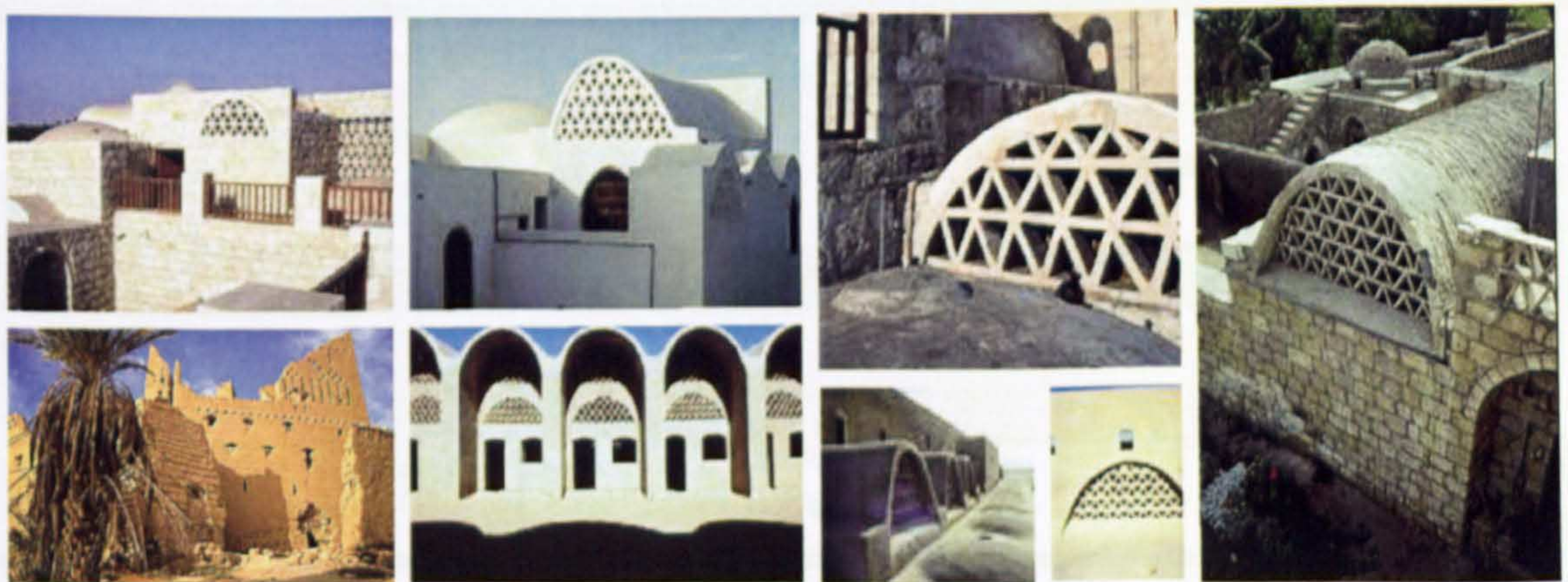
Figure 3-6 Photos Depicting Doubled Roof and Roofs Vents
