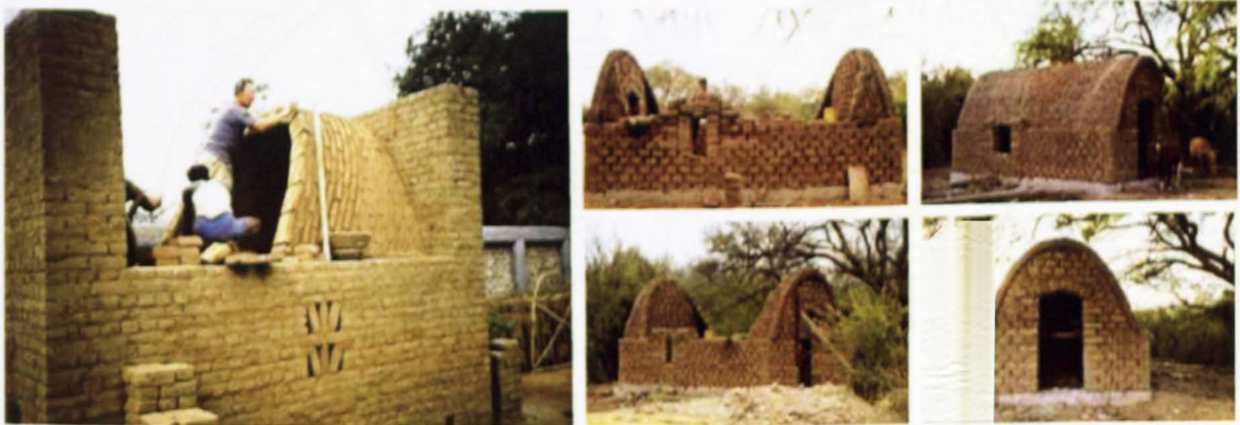
Figure 4-5 The Nubian Way for Erecting Vaults, Source: www.canellect.com [14]
