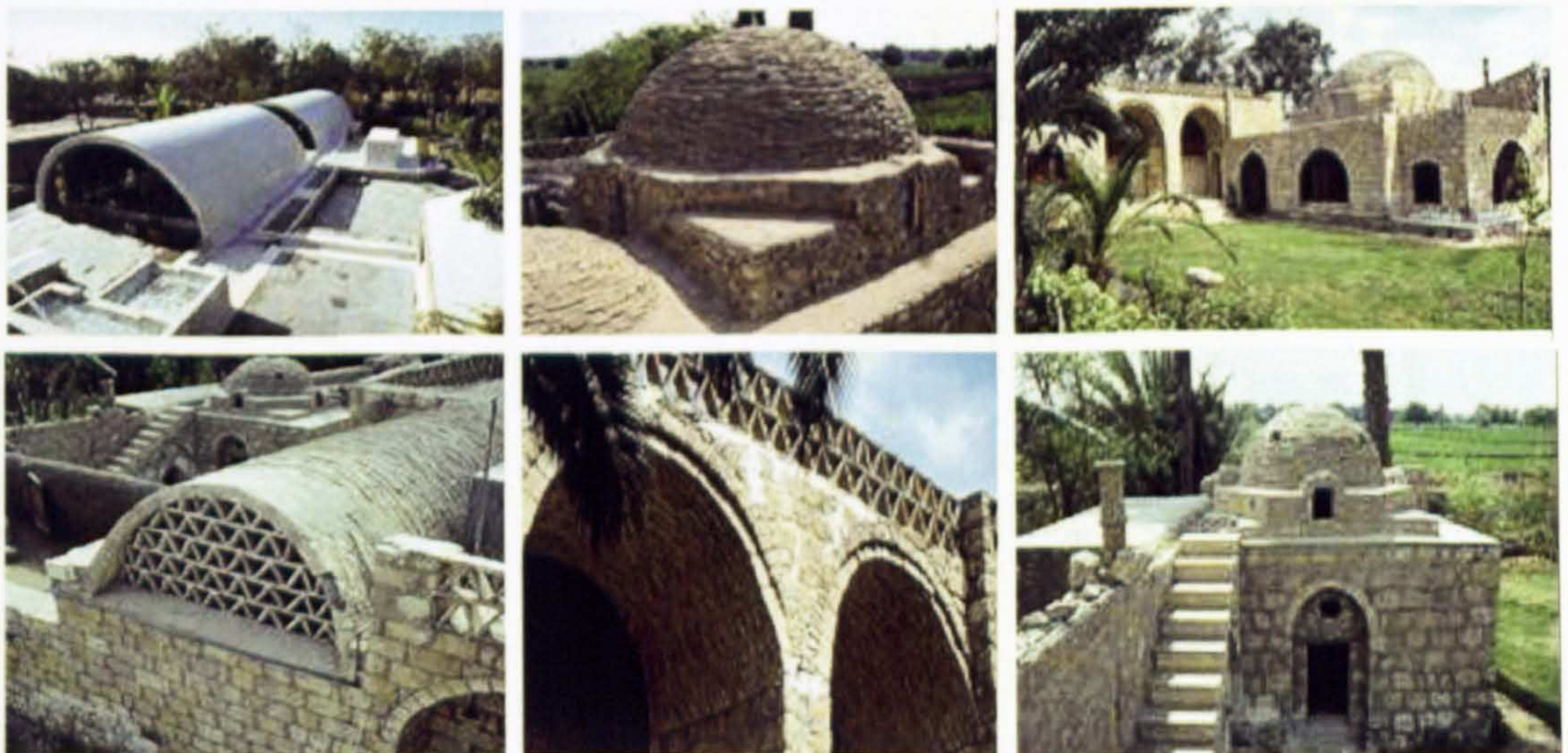
Figure 3-3 Different Shapes of Contemporary Curved Roofs
