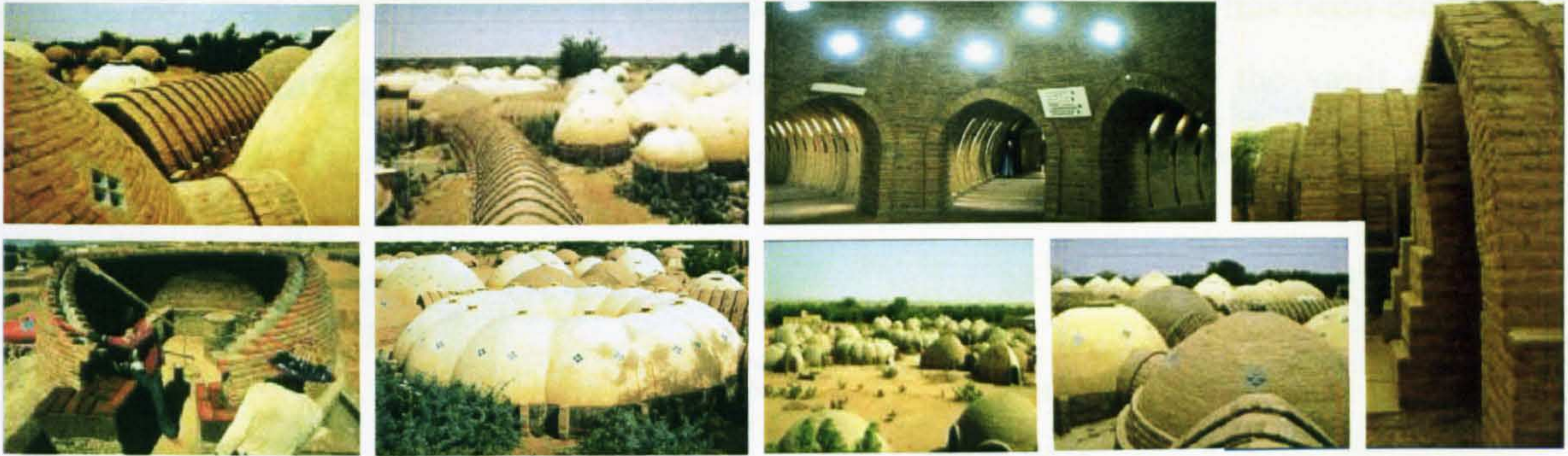
Figure 4-27 The Regional Hospital, Mauritania Source: ArchNet Digital Library [13]
