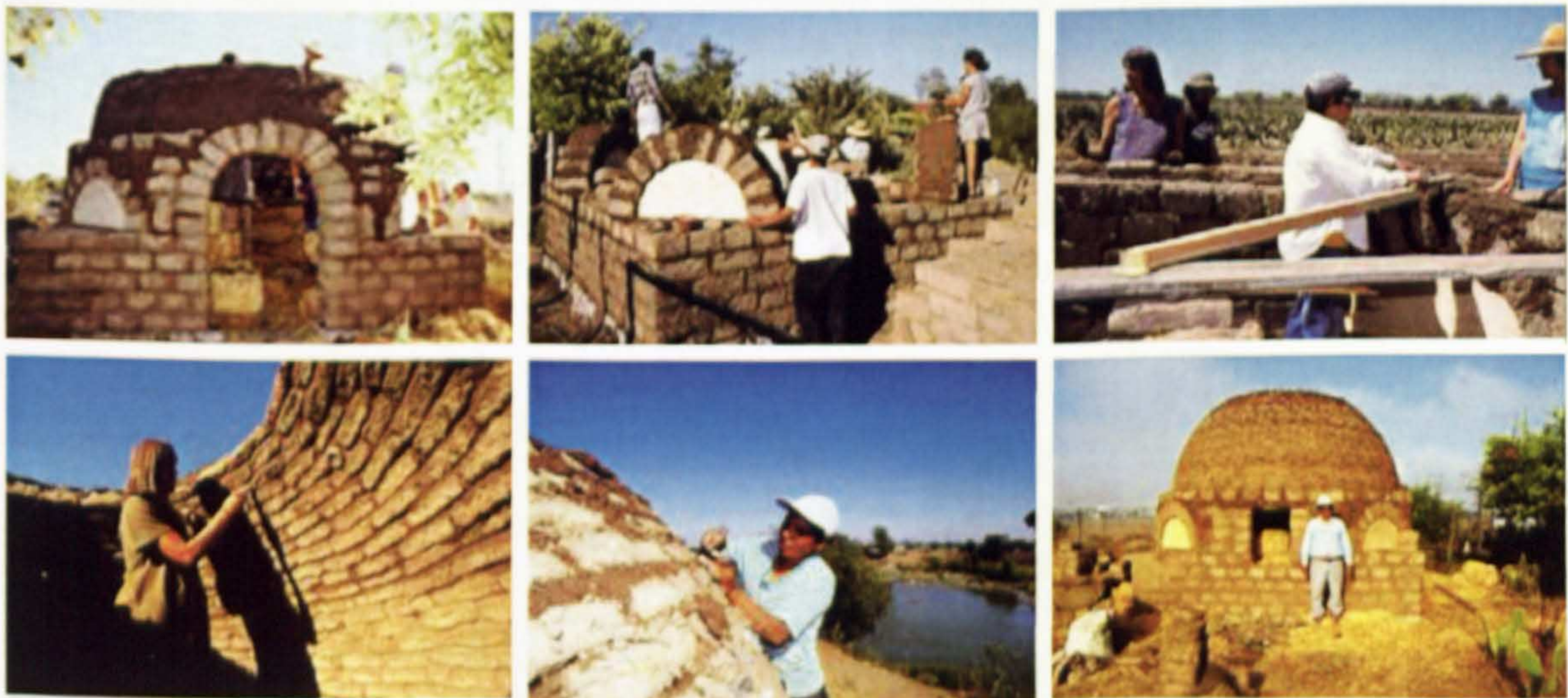
Figure 4-11 Woodless Stones and Mud Bricks Domes on Pendentives
