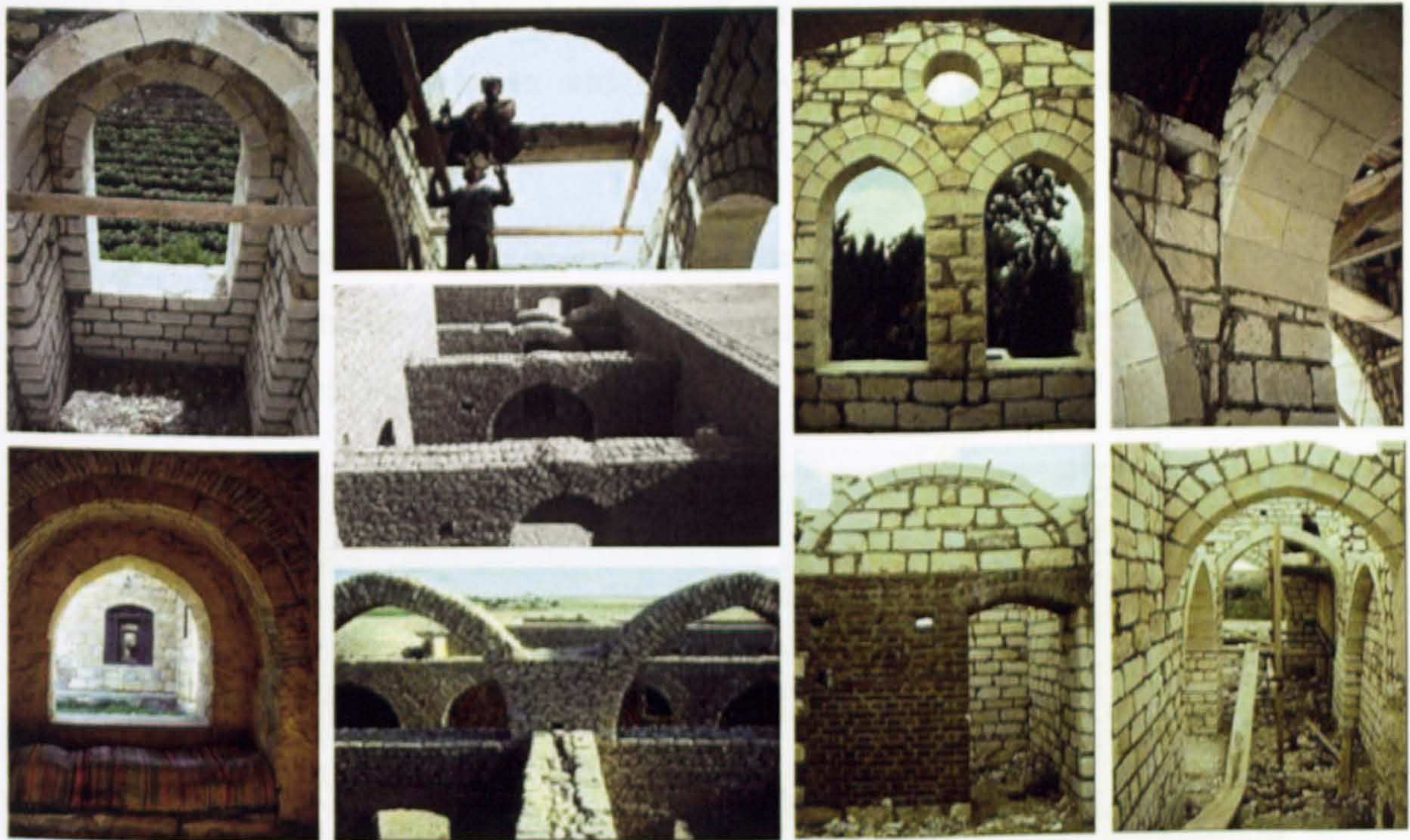
Figure 4-12 Woodless Bricks and Stones Constructions in Southern Part of Egypt Source: ArchNet Digital Library [13]
