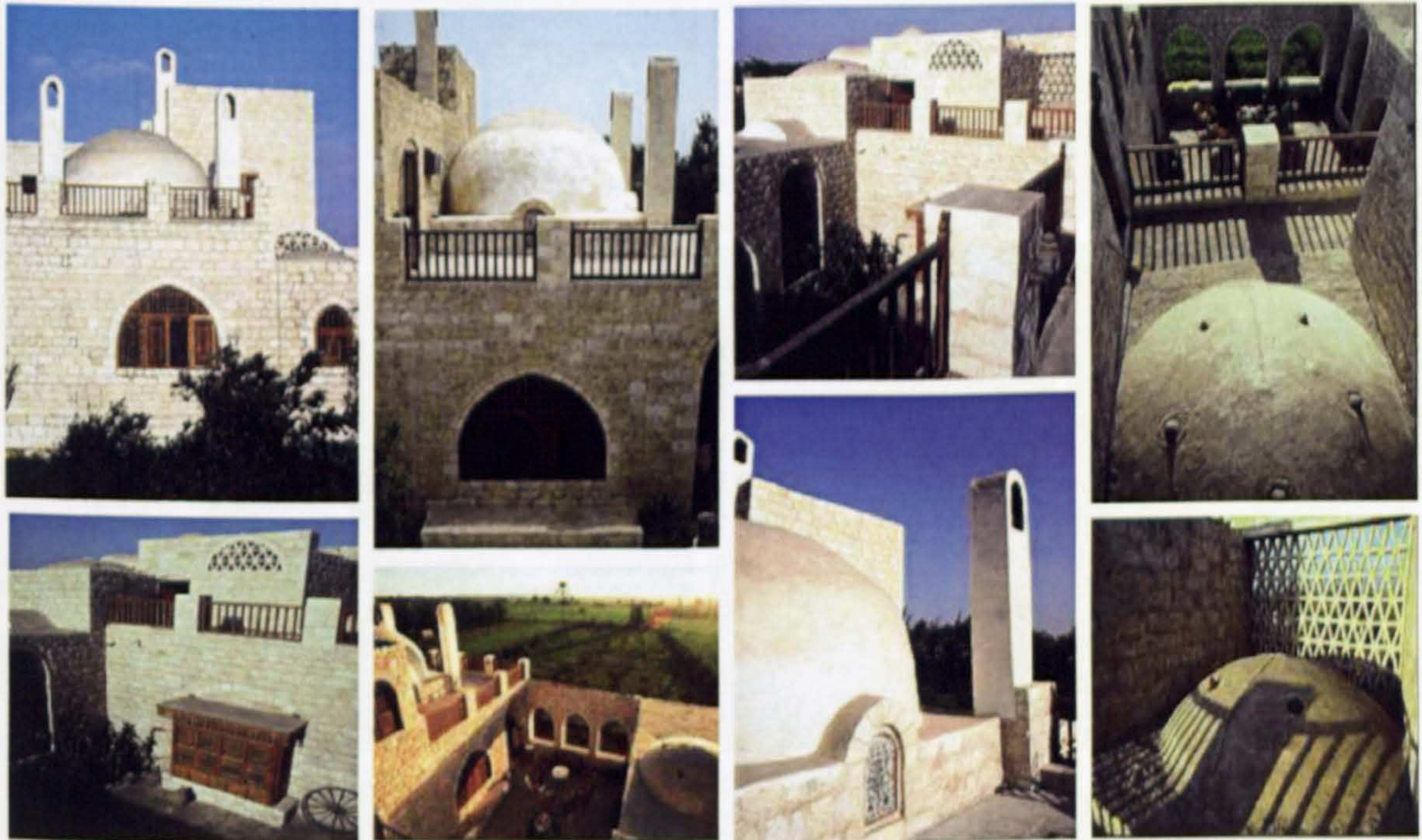
Figure 4-20 Casaroni House (Exterior), Source: ArchNet Digital Library [13]
