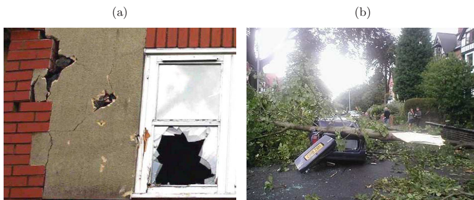
Figure 1.4: Damage to (a) building facades (Marshall and Robinson, 2006) and (b) cars due to windborne debris generated during the 2005 Birmingham Tornado (BBC, 2005).
