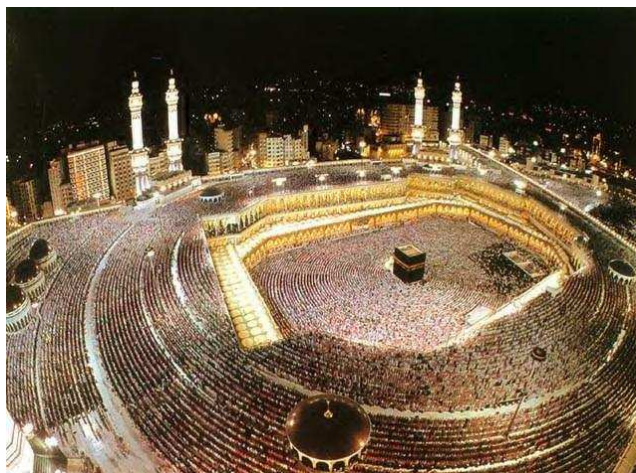
Figure 6. 18. Mekkah Holy Mosque in Saudi Arabia (Source: http://media.isnet.org/iptek/100/ )
