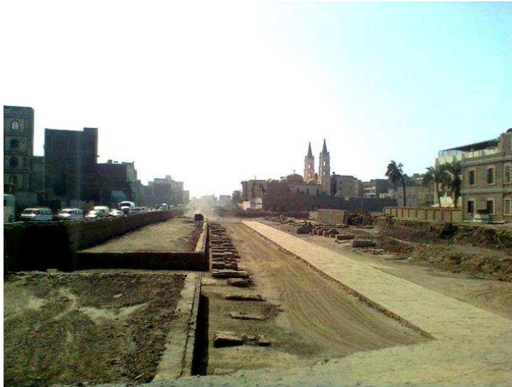
Figure 7. 3. The Avenue of Sphinxes' excavations
