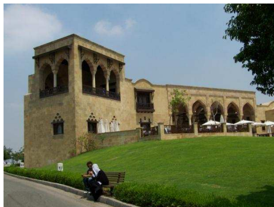
Figure 4. 27. The use of traditional takhtaboush opened to exterior and the use of characterized Fatimid arches.
