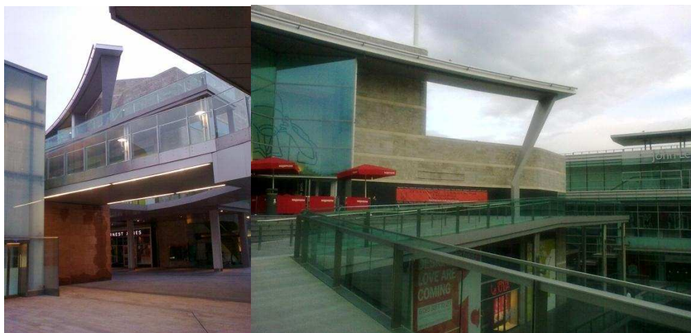
Figure 5. 18. Masses, bridges and metalwork canopy- an analogy of the Old Dock
