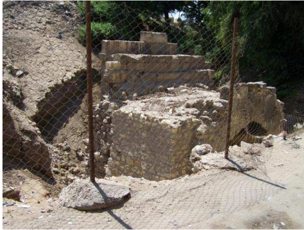
Figure 7. 1. An example of physically inappropriate heritage sites, a part of Historic Cairo's Saladin's Wall- the remains are un-restored, fenced and with no access
