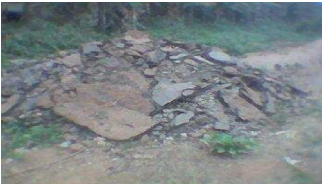
Figure 2.3a: Ripped Asphalt Improperly Disposed Close to Farmland along Igede - Aramoko Road in Ekiti State, Nigeria
