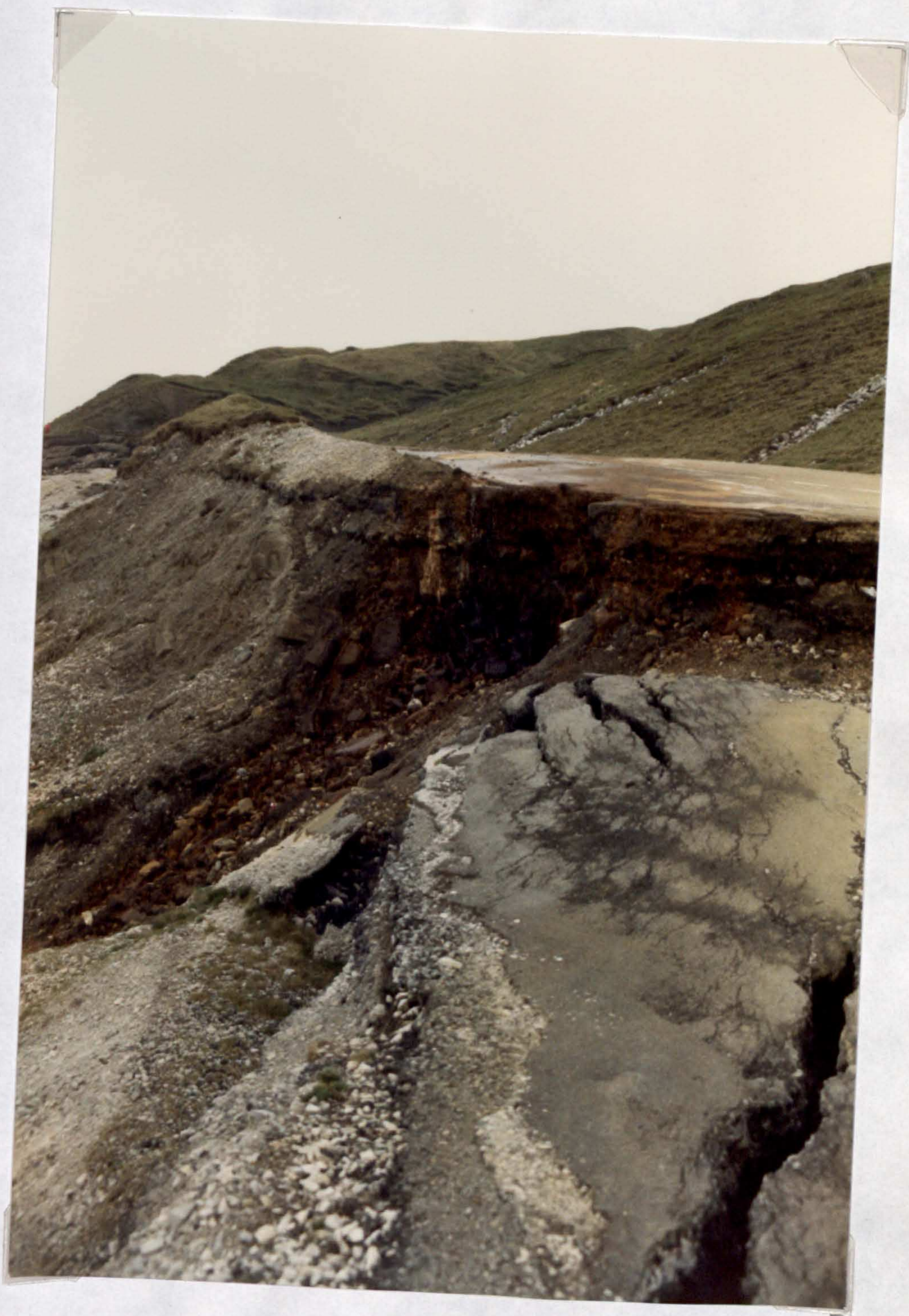
PLATE 6.2 OCHREOUS PRECIPITATE AT MAM TOR LANDSLIDE
